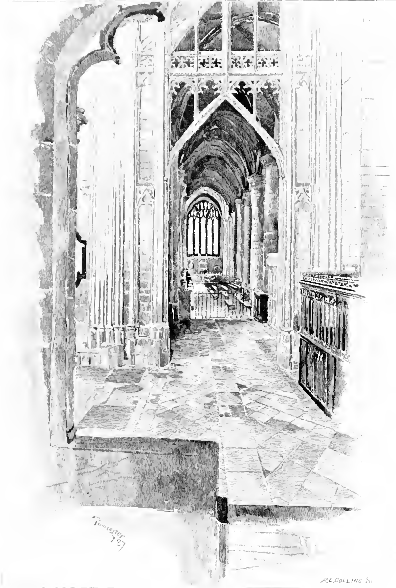
THE SOUTH AISLE OF THE NAVE, LOOKING WEST FROM THE TRANSEPT.
