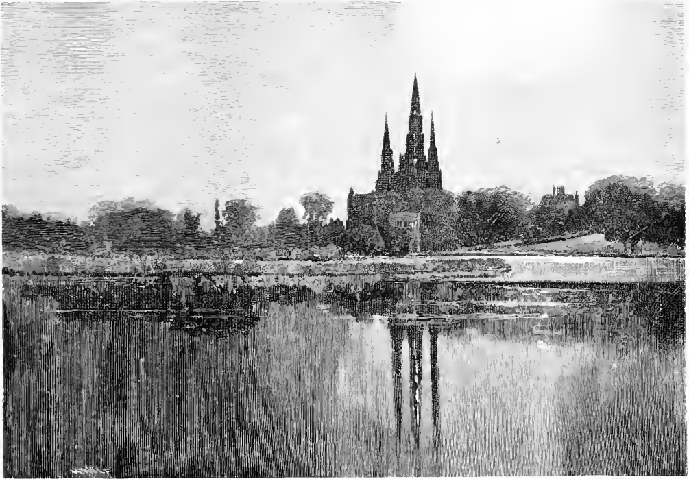
LICHFIELD CATHEDRAL, FROM THE EAST.
