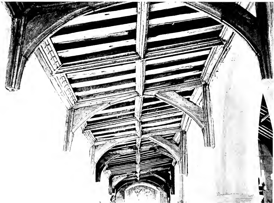
SOUTHACRE, NORFOLK, FLYING BUTTRESS ROOF OF AISLE
