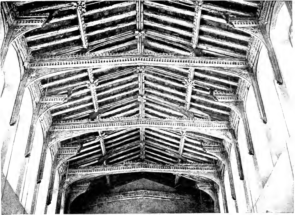
WALSHAM-LE-WILLOWS, SUFFOLK, INTERMEDIATE HAMMER-BEAM PRINCIPALS
