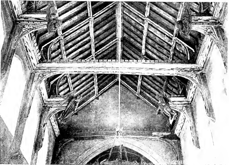
UFFORD, SUFFOLK, INTERMEDIATE HAMMER-BEAM PRINCIPALS
