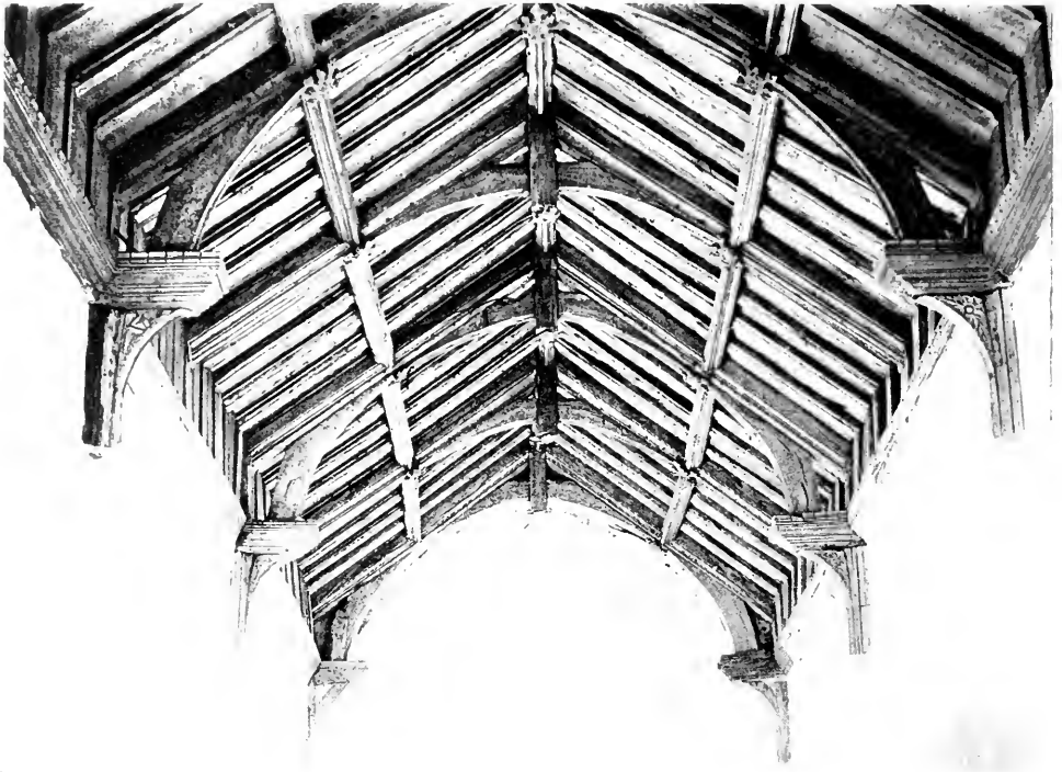
SOUTHACRE, NORFOLK, HAMMER-BEAM ROOF OF NAVE
