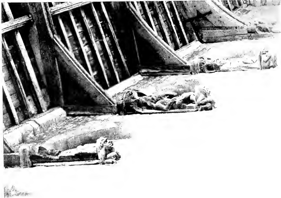
WHISSENDINE, RUTLAND, ROOF OF NAVE
