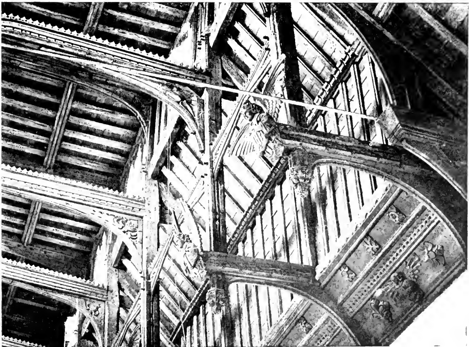
NEEDHAM MARKET, SUFFOLK, DETAIL OF ROOF
