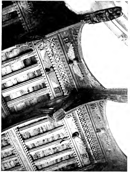
EARL STONHAM, SUFFOLK, CORNICE
