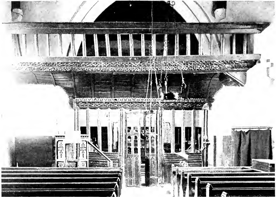
LLANEILIAN, ANGLESEY, OPEN PANELS WITHOUT TRACERY
