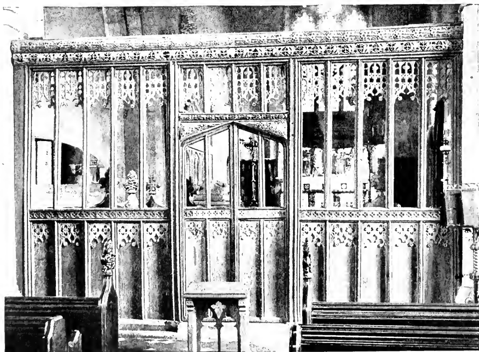
BACKWELL, SOMERSET, MULLIONS RUN THROUGH TO HEAD
