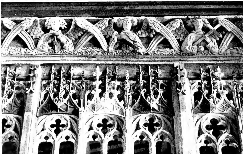
HITCHIN, HETS., TRACERY WITH APPLIED TABERNACLE WORK
