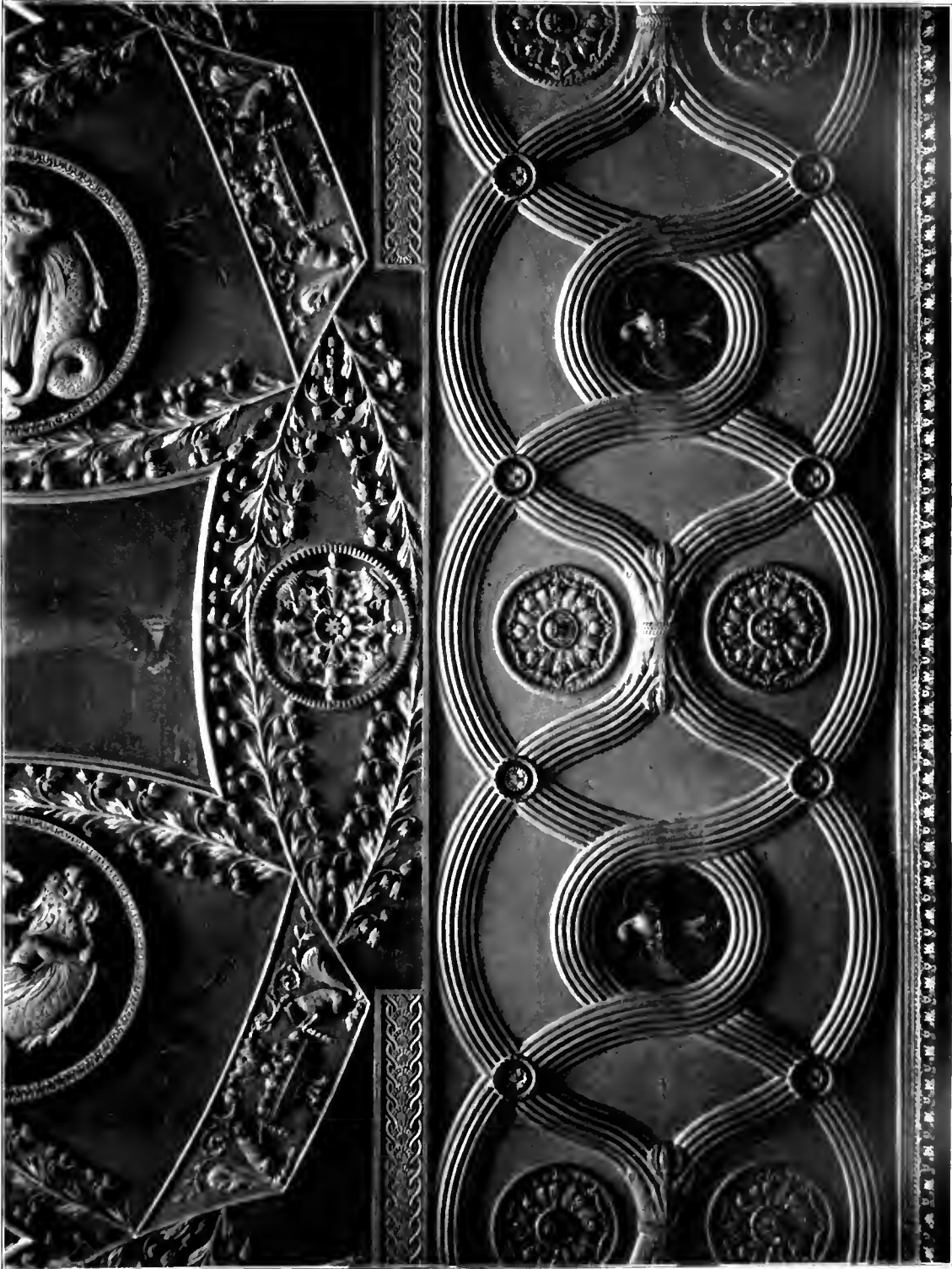
Portion of a Ceiling, consisting of painted panels and moulded plaster. From Nr. 15 Hanover Square, London, Late 18 th Century The original paintings with reproductions of the plaster work are now in the Victoria and Albert Museum
