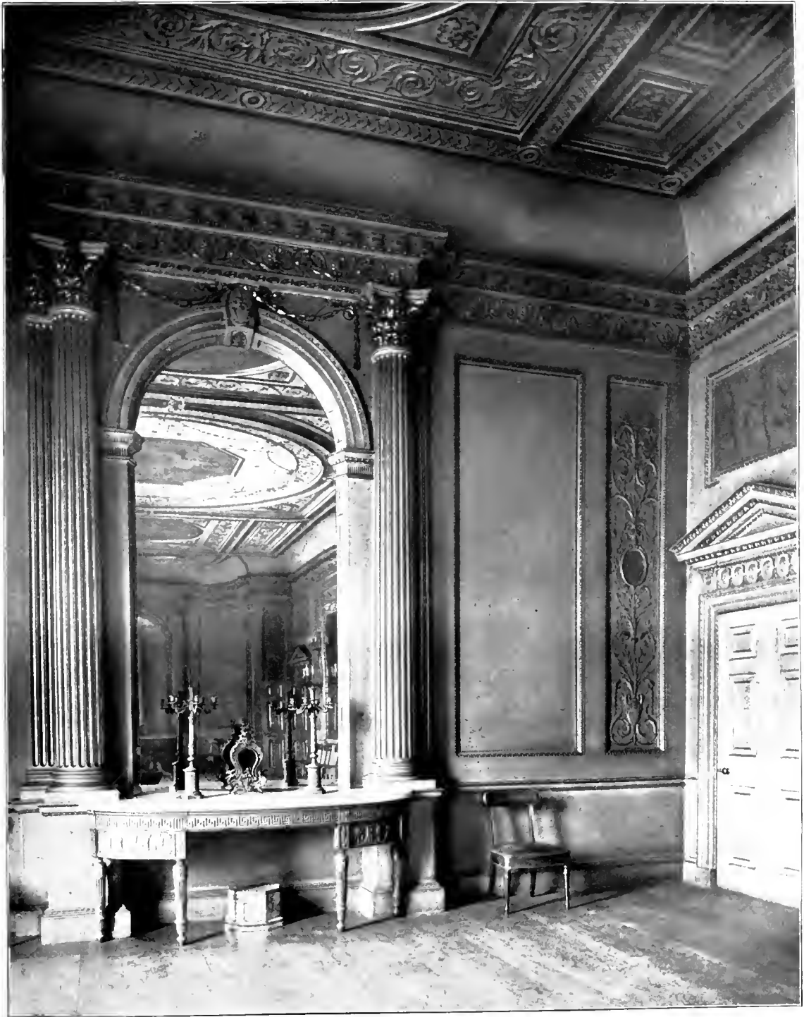
Carrington House, Whitehall. Ball Room by Sir William Chambers, about 1760; now pulled down
