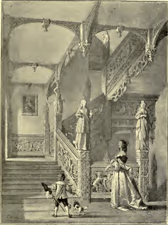
STAIRCASE, ALDERMASTON, BERKSHIRE.
