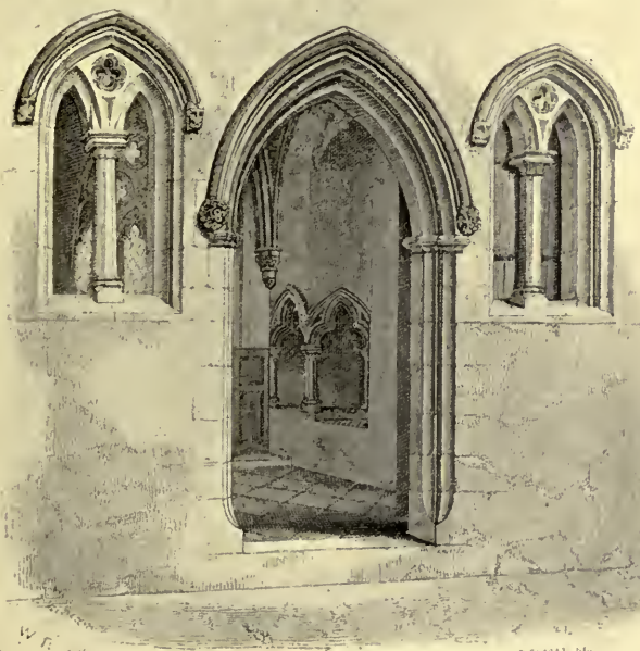
CHAPEL ENTRANCE, LITTLE WENHAM HALL, SUFFOLK
