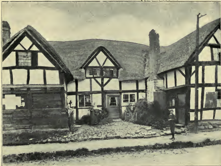
COTTAGES AT KINGSLAND, HEREFORDSHIRE.
