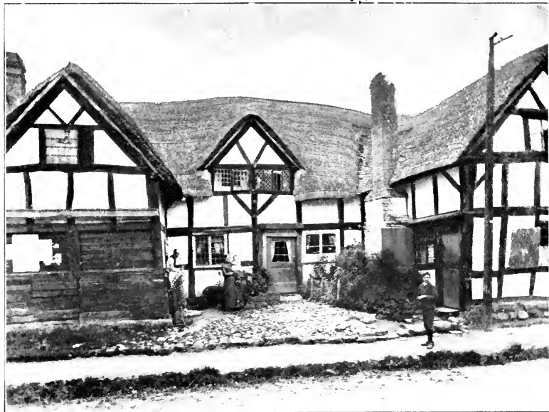
COTTAGES AT KINGSLAND, HEREFORDSHIRE.
