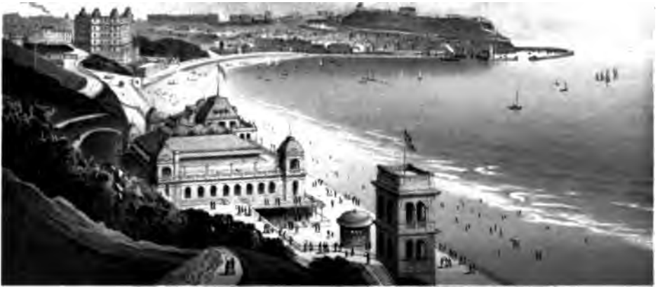
THE SOUTH BAY — STARBUROUGH
