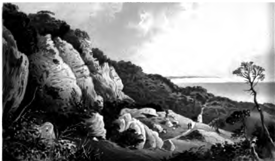
THE LANDSLIP NEAR VENTNOR— ISLE OF WIGHT.
