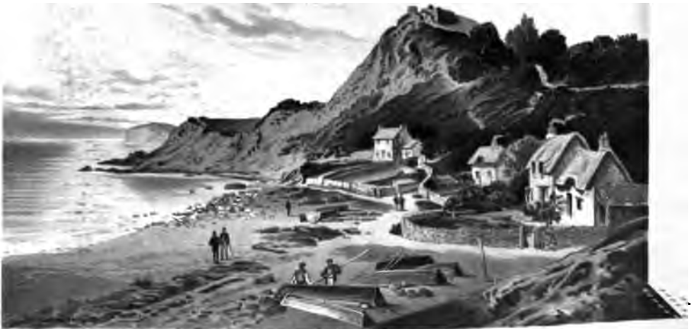
STEEP MILL COVE, VENTNOR - ISLE OF WIGHT
