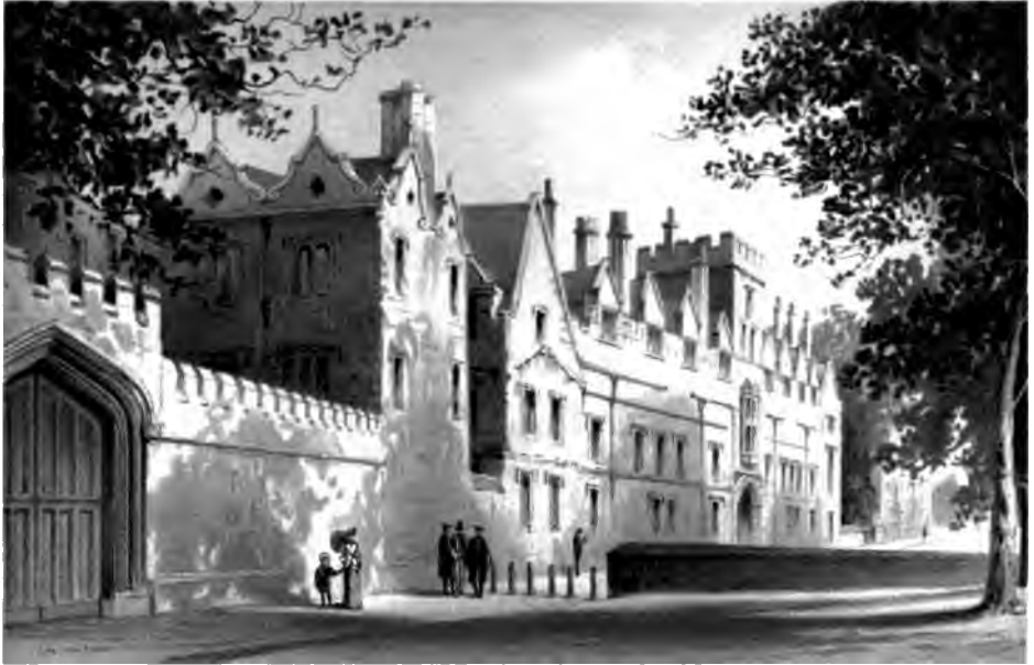
View of the building from the left
