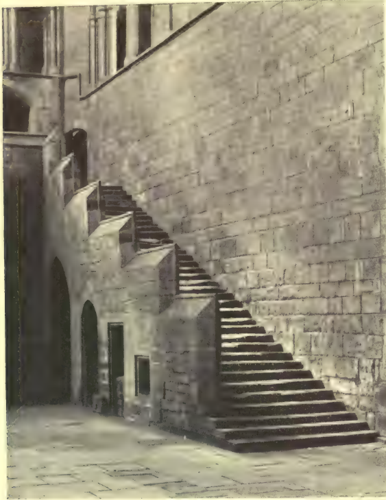
Fig. 1. STAIR TO THE DORMITORY, HEXHAM PRIORY.
