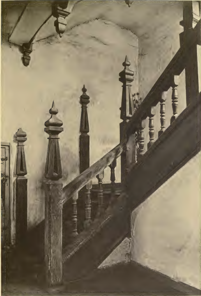
ASTON BURY, HERTFORDSHIRE. SECOND STAIR.
