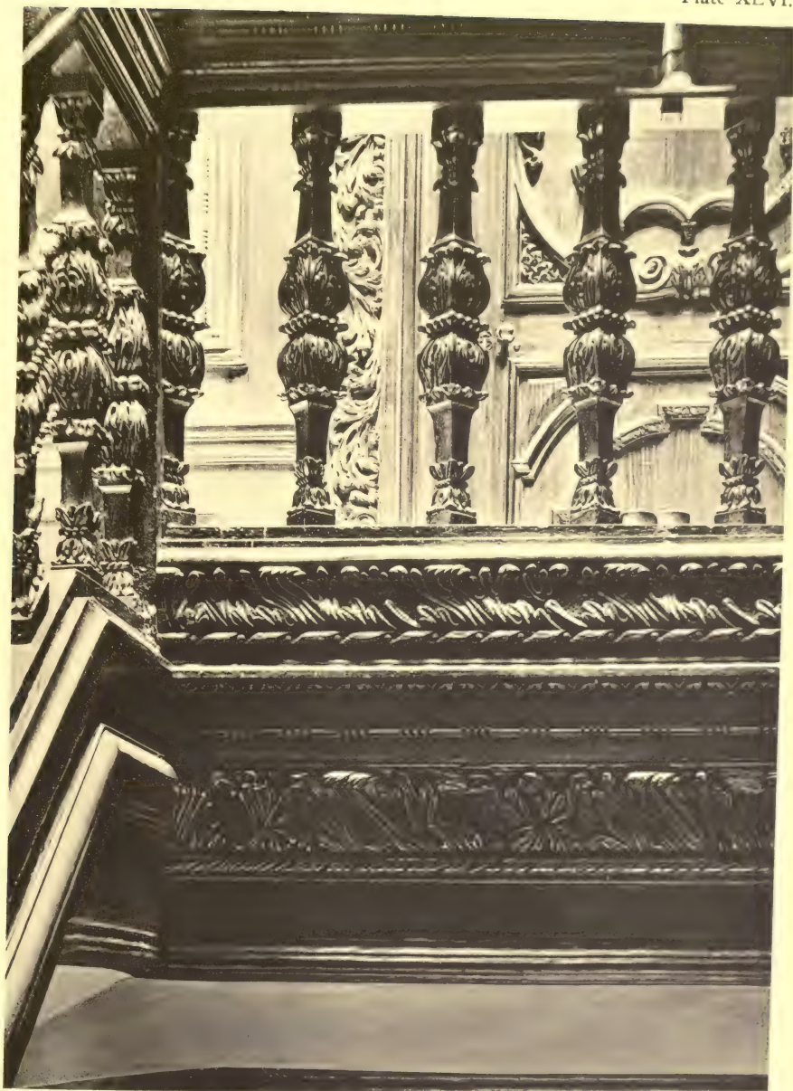
HOPETOUN HOUSE, SCOTLAND. DETAIL OF BALUSTERS AND STRING.
