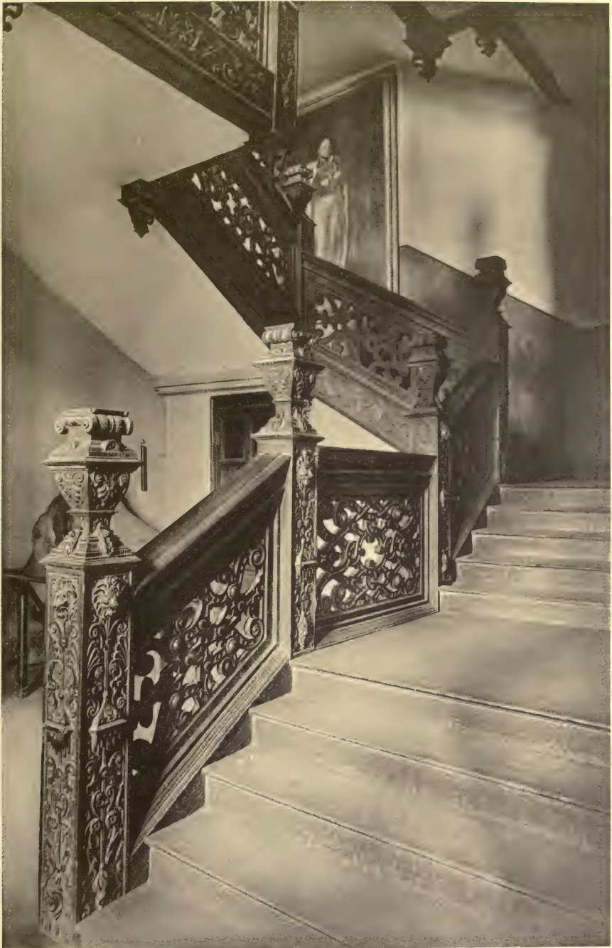
ASTON HALL (1618-35), WARWICKSHIRE.
