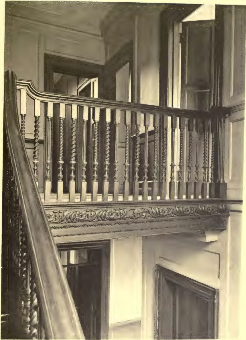
FRIENDS' HOUSE, CROYDON, SURREY. UPPER LANDING.
