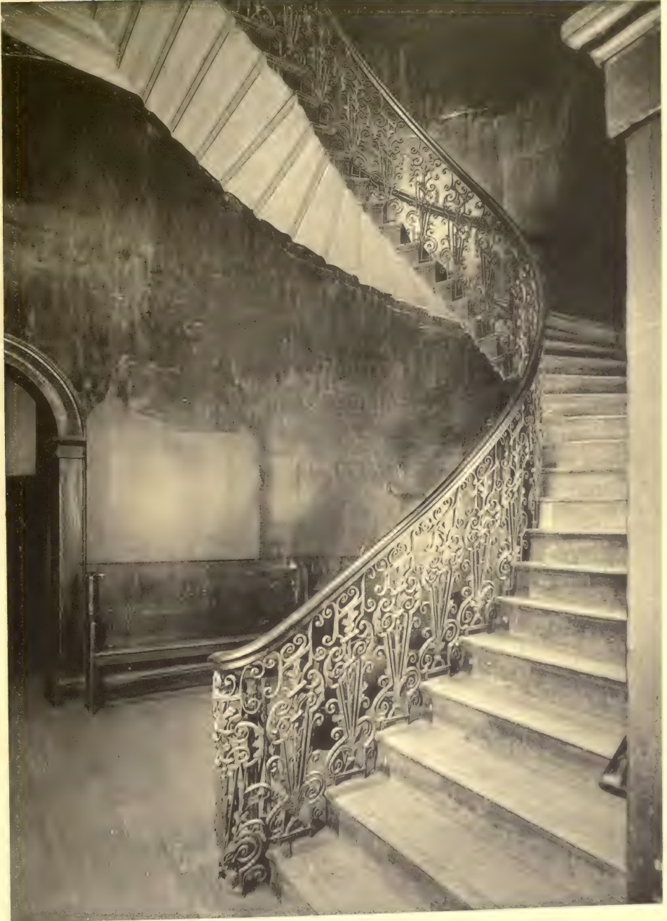
NO, 35, LINCOLN'S INN FIELDS, LONDON. LOWER STAIR RAIL.
