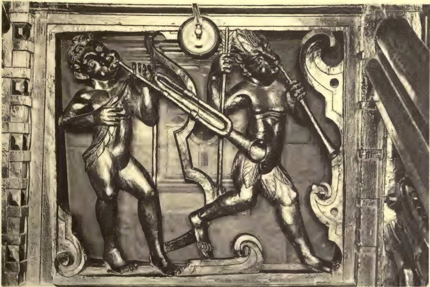
CARVED PANELS ON STAIRCASE AT RAWDON HOUSE, HODDESDON. (1622.) SUBJECTS: "SAMSON AND DELILAH," AND "MUSICIANS."
