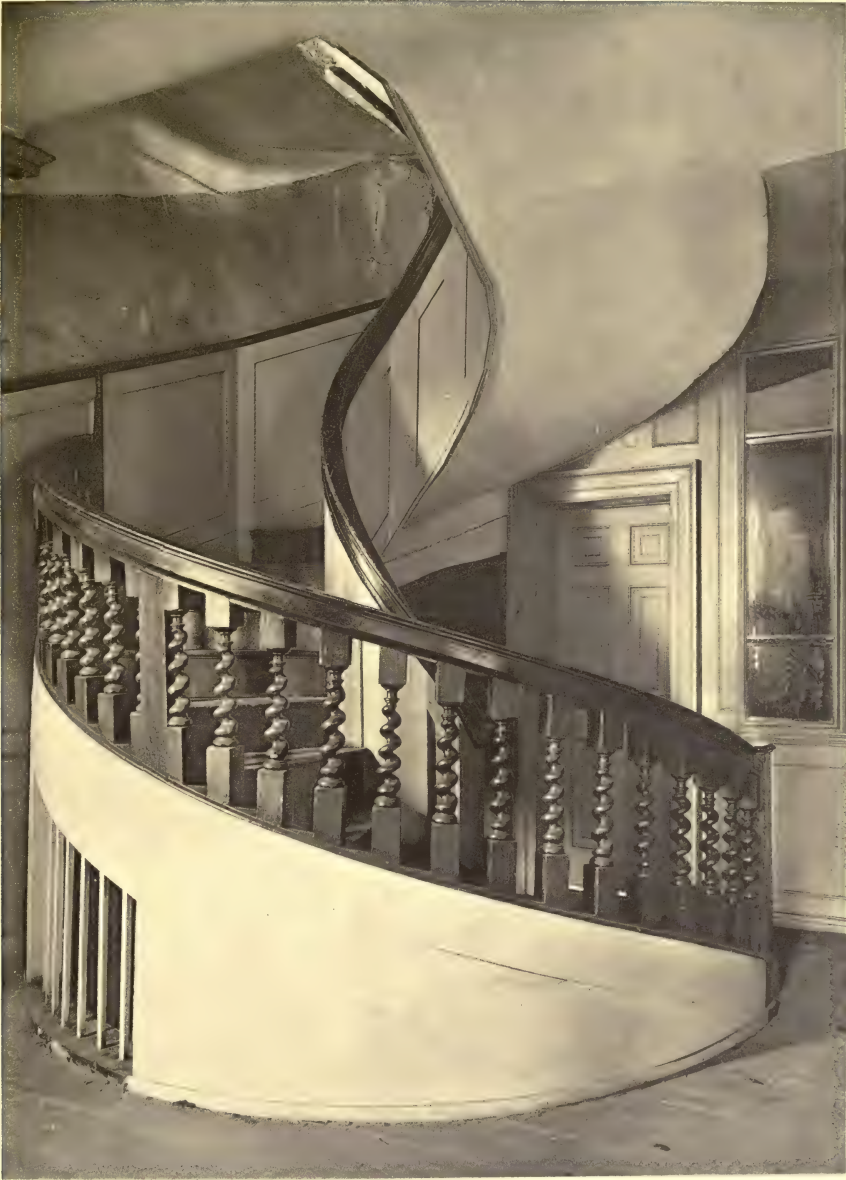
THE FRIARS, AYLESFORD. CIRCULAR STAIR.
