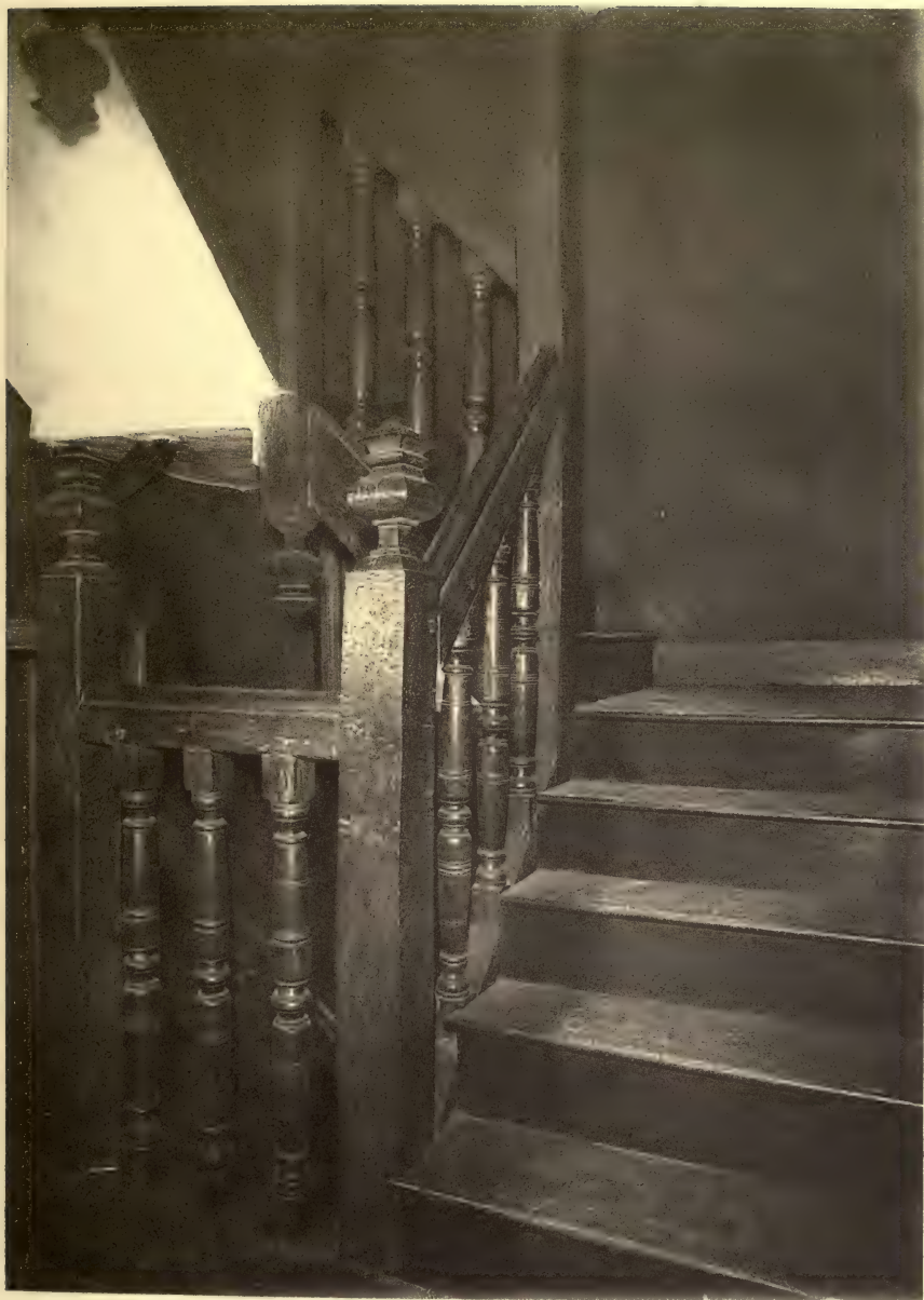
RESTORATION HOUSE, ROCHESTER, UPPER STAIR.
