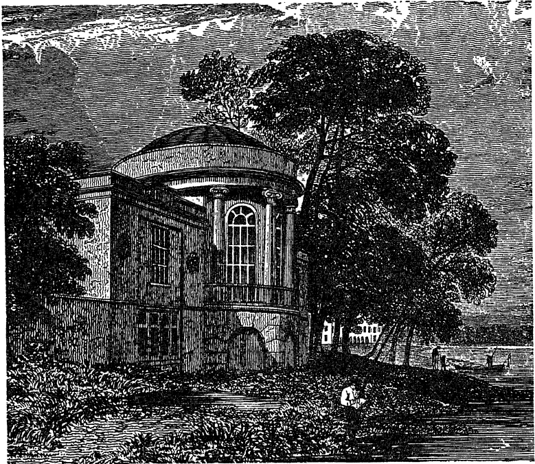
The Duke of Northumberland's boathouse on the Thames near Syon House, Middlesex. This small, graceful structure, often wrongly attributed to Robert Adam, was designed by James Wyatt, who had a comparable delicacy of touch when handling the classic idiom. From a drawing by J. D. Harding, engraved by W. B. Cooke, and included in Barbara Hofland's Richmond and its Surrounding Scenery (London: 1832).
