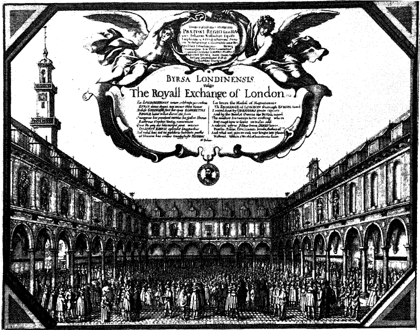
PLATE 27. The Royal Exchange, London, founded by Sir Thomas Gresham (1519–1579), and one of the first buildings to be entirely Flemish in style, for the work was commissioned in Flanders by Gresham, and the master-mason who carried it out was a Fleming named Henryk. The principal feature of the building was a great courtyard, surrounded by a loggia, with the arches supported on Doric columns, and Ionic pilasters on the upper storey between the niches. The two orders were used with clarity and decision, undistorted by the fanciful additions that often characterised Flemish interpretations of classic architecture. This building may well have exerted an influence on English architects who were experimenting with the use of the classic orders. It was begun in 1566, opened by Queen Elizabeth I in January 1571, and destroyed by fire in 1666. This view is from an engraving by Hollar, 1644. Reproduced by courtesy of the Trustees of the British Museum.
