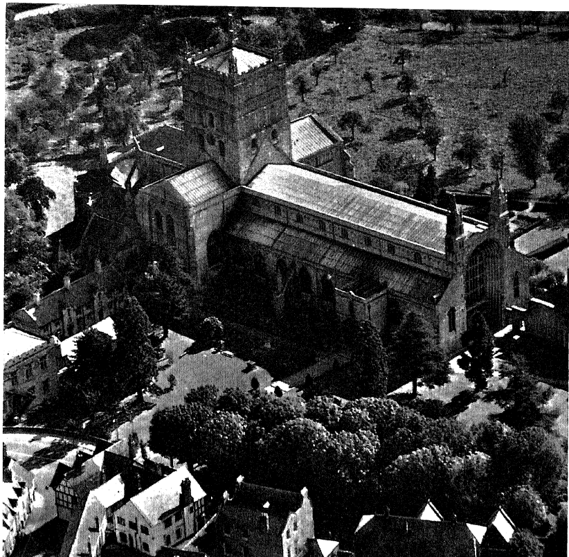
PLATE 7. The Abbey Church of Tewkesbury, Gloucestershire, consecrated in 1125. An example of early Norman work, this cruciform structure has a nave with side aisles, transepts, and a choir terminating in an apse, surrounded by an ambulatory. Nave, choir and transepts are united by a central tower, 46 feet square and rising to 135 feet: the largest Norman tower in Europe. (The rich arcading of the tower is shown in the drawing on page 44.) The west front is dominated by a huge arch, which streams upwards to the roof line. Norman work still gives a bold, massive character to the interior, although the church was restored in the Decorated period. Unlike Buildwas (plate 6), Tewkesbury survived: when the Abbey was suppressed in 1540, the Abbey Church was bought from the King's Commissioners by the people of Tewkesbury, and it became their parish church. Photograph by Aerofilms.
