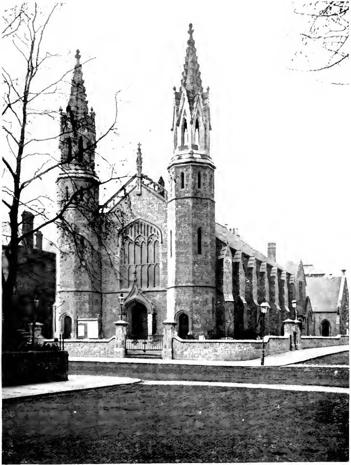
CAMDEN ROAD BAPTIST CHURCH, LONDON. (Photo: F. Thurston, F.R.P.S., Luton.)
