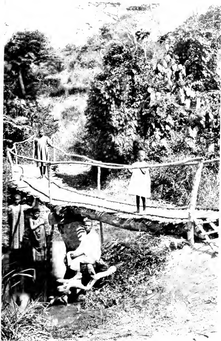
BRIDGE OVER L'USENGELE STREAM NEAR COMBER STATION, KIBOROLO.
