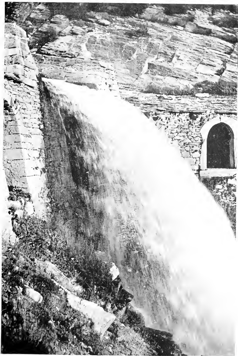
RUNNING BENEATH AVALANCHE GALLERIES THE SIMPLON PASS
