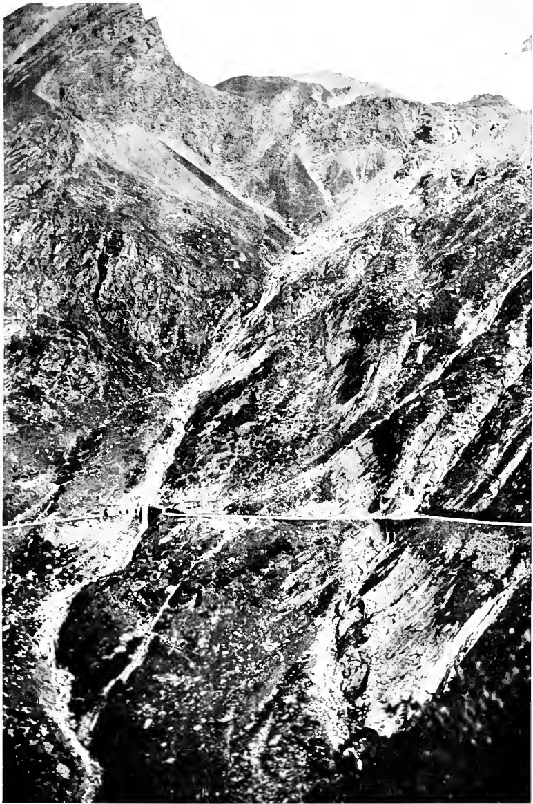
THE ROAD CLINGS TO THE MOUNTAIN SIDE THE STAPLON PASS
