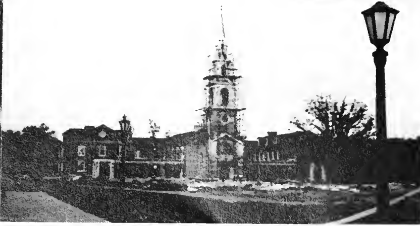
Work on the Steeple.
