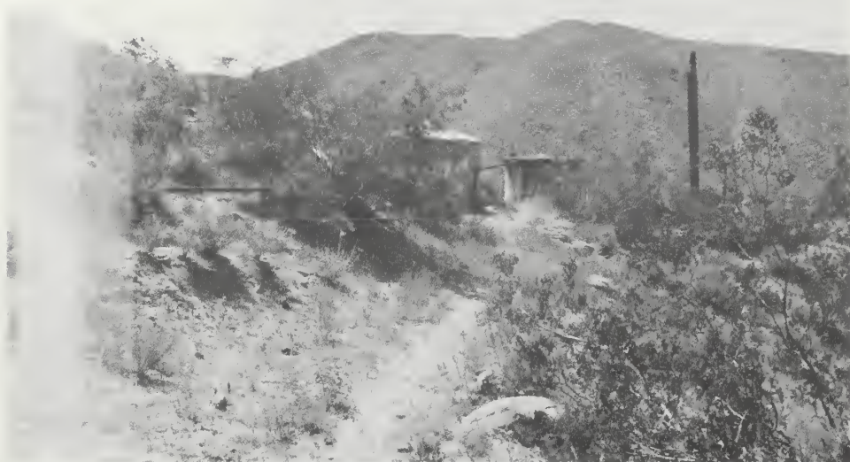
(a) Tanks used to store water piped from Alpha Springs.
