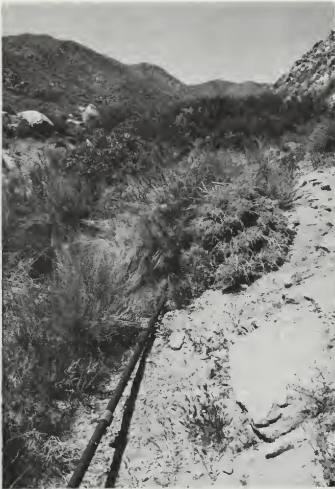
(a) Pipeline diverting water from Benko Spring.
