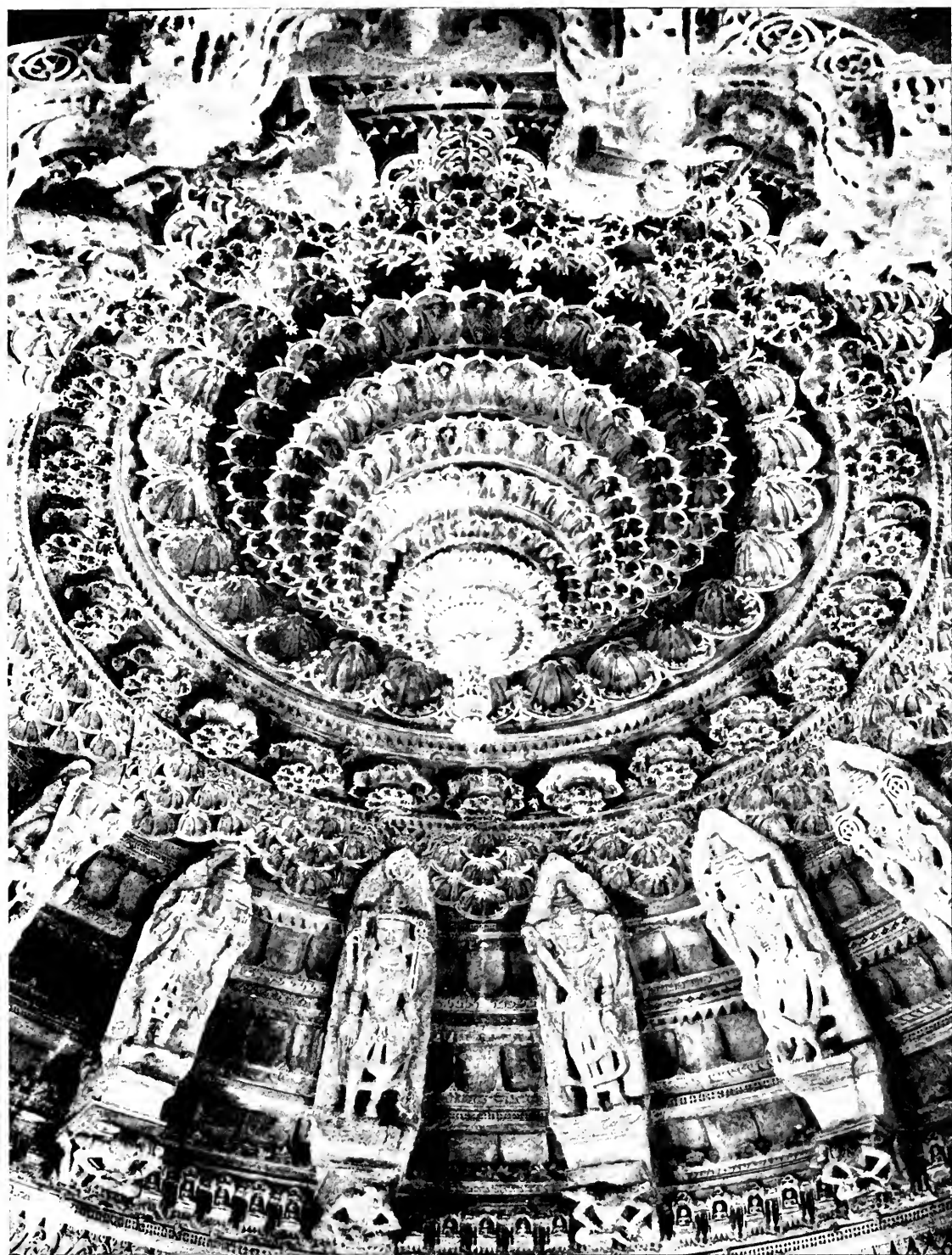
Ceiling Work in Dilwara Temples (Mt. Abu).
