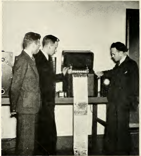
This facsimile machine is a device for printing pictures as received from the broadcasting station via the radio waves. Every evening after the regular broadcast is over a Philadelphia station presents this service and Lehigh has been quite willing to use it.
