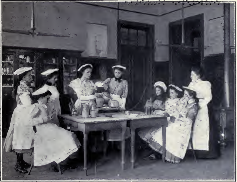
Fig. 44. Equipment in Elementary Public School, Washington, D. C.
