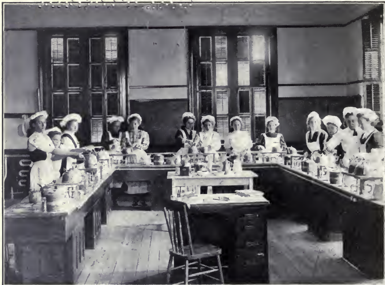
Fig. 46. Kitchen remodeled from classroom, Tenafly, N. J.
