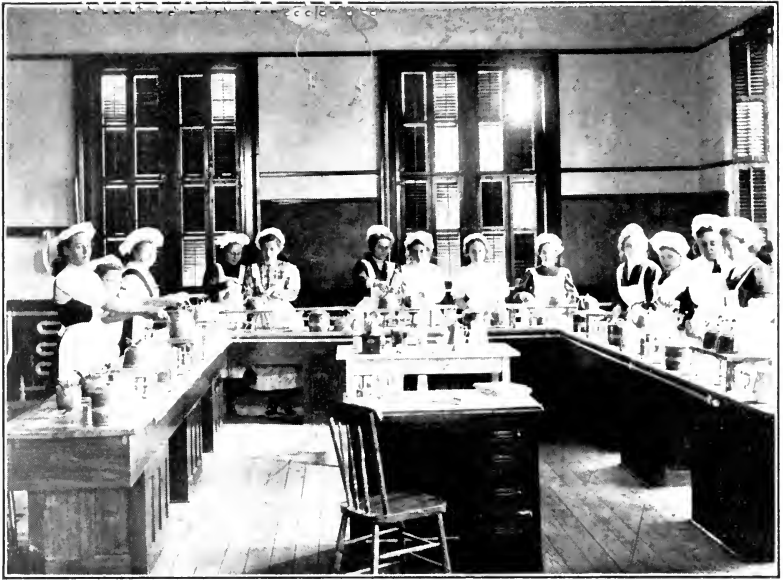
Fig. 46. Kitchen remodeled from classroom, Tenafly, N. J.
