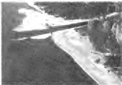
Figure 18. An aerial view of the silt accumulating in the Ohio River at the mouth of the Post Creek Cutoff
