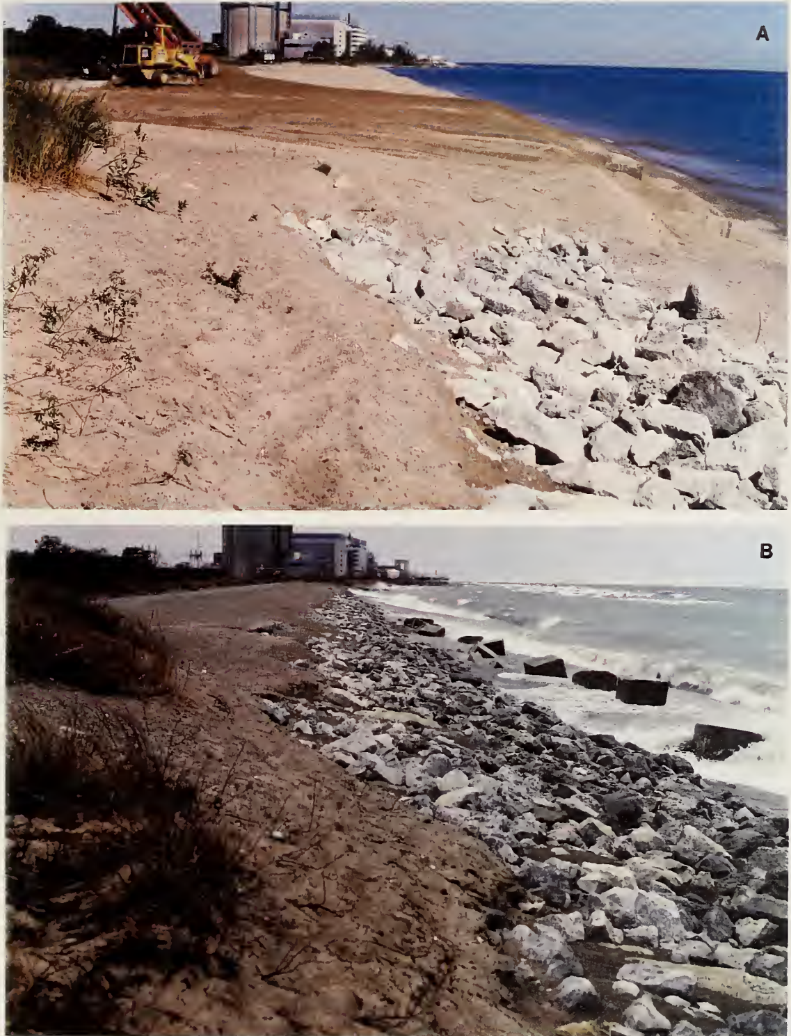
Figure 3-16 Photographs showing the IBSP/SU beach-nourishment stockpile. Photographs show stockpile geometry: (A) just prior to completion of 1997 nourishment; and (B) eight weeks following nourishment. View is to the north. Note that concrete cubes and riprap are re-exposed in (B) due to erosion of nourishment material (photo dates: September 17, 1997 (A), and November 14, 1997 (B)).
