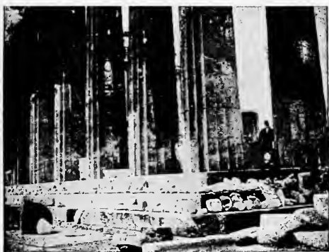
FIG. 13.—PHOTOGRAPHIC EFFECT OF CURVED STYLOBATE AND COLUMN OF THE PARTHENON.
