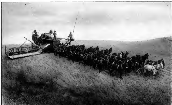
FIG. 3. A modern wheat-heading-and-threshing machine
