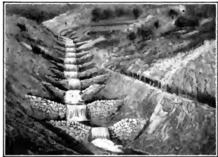
Working to prevent erosion after the removal of the forest in the French alps.
