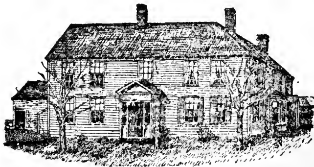
MOSES BOYNTON HOUSE.
