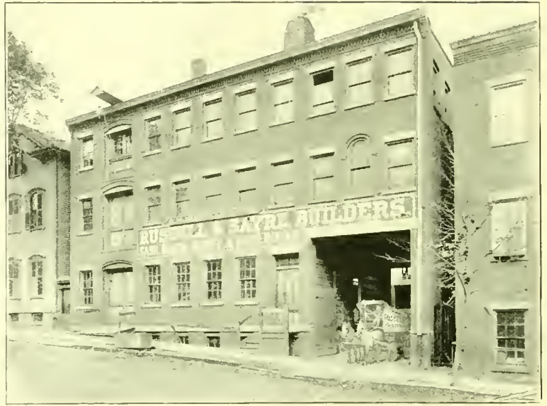
WORKS OF C. M. RUSSELL, BUILDER, 38 AND 40 CRAWFORD STREET.
