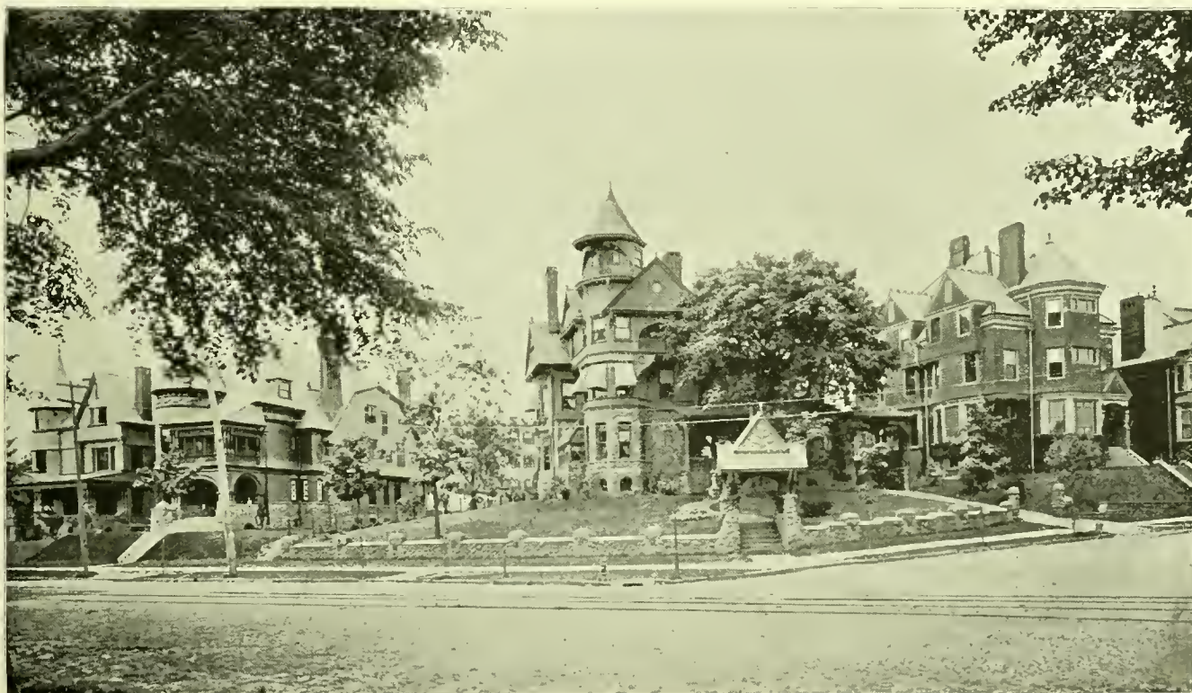
VIEW ON CLINTON AVENUE AND HIGH STREET, NEWARK, N. J.
