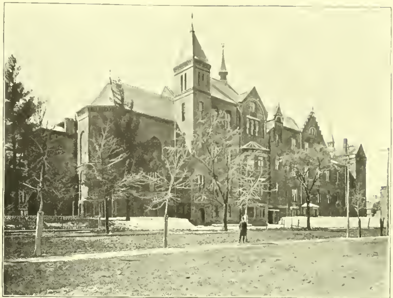
ST. BARNABAS HOSPITAL, HIGH AND MONTGOMERY STREETS.
