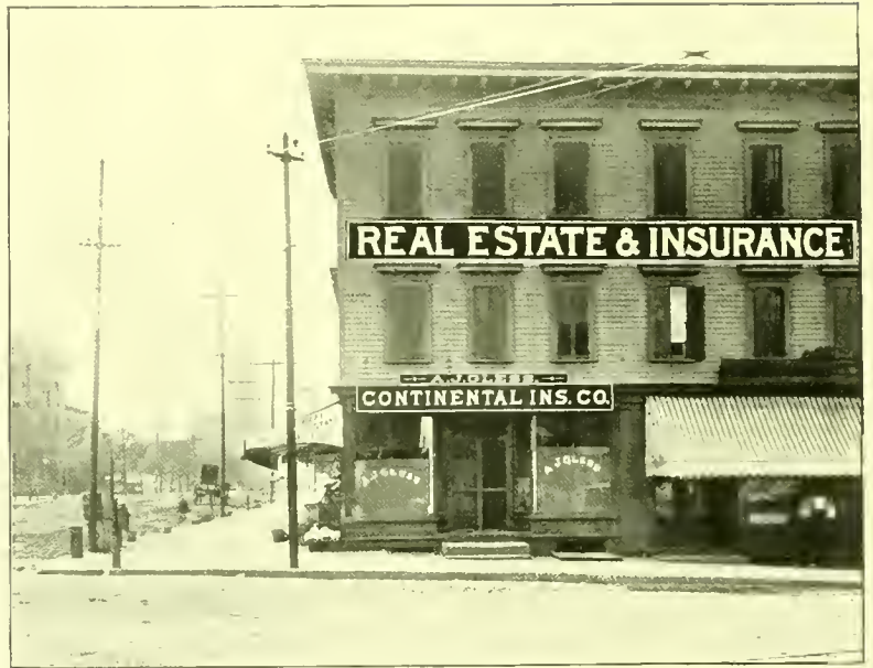
OFFICE OF A. J. GLESS, CORNER SPRINGFIELD AND BELMONT AVENUES.
