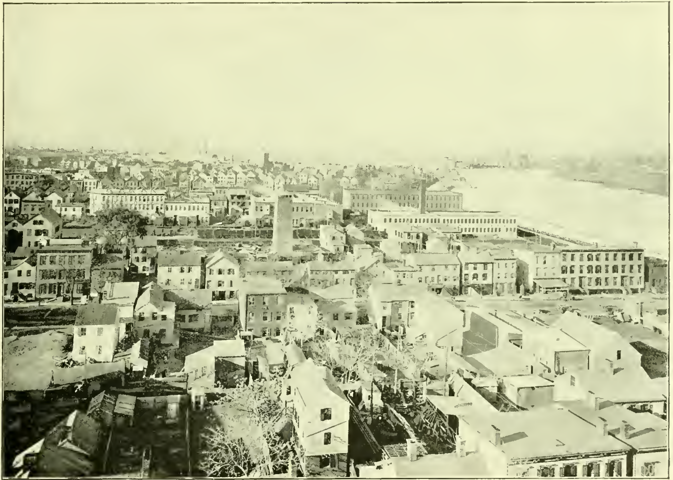
VIEW IN NEWARK, N. J., LOOKING NORTHWEST FROM FREEMAN STREET.
