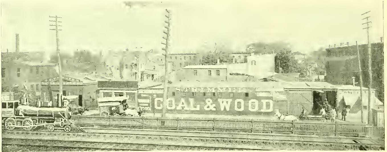
COAL AND WOOD YARD OF S. TRIMMER & CO., CORNER NEW JERSEY RAILROAD AVENUE AND LAFAYETTE STREET.
