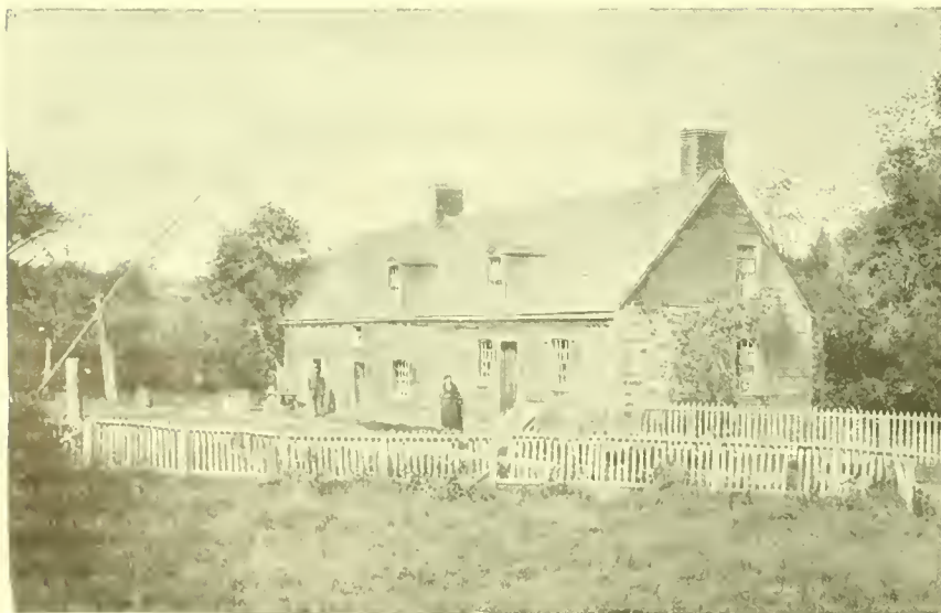
MEEKER HOMESTEAD, THE OLDEST LANDMARK IN ESSEX COUNTY, N. J.
