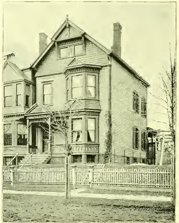
RESIDENCE OF LOUIS A. FELDER, ON LITTLETON AVE.
