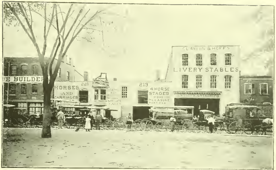
THE CLAYTON-HOFF CO., LIVRY STABLES, ON HALSEY STREET.
