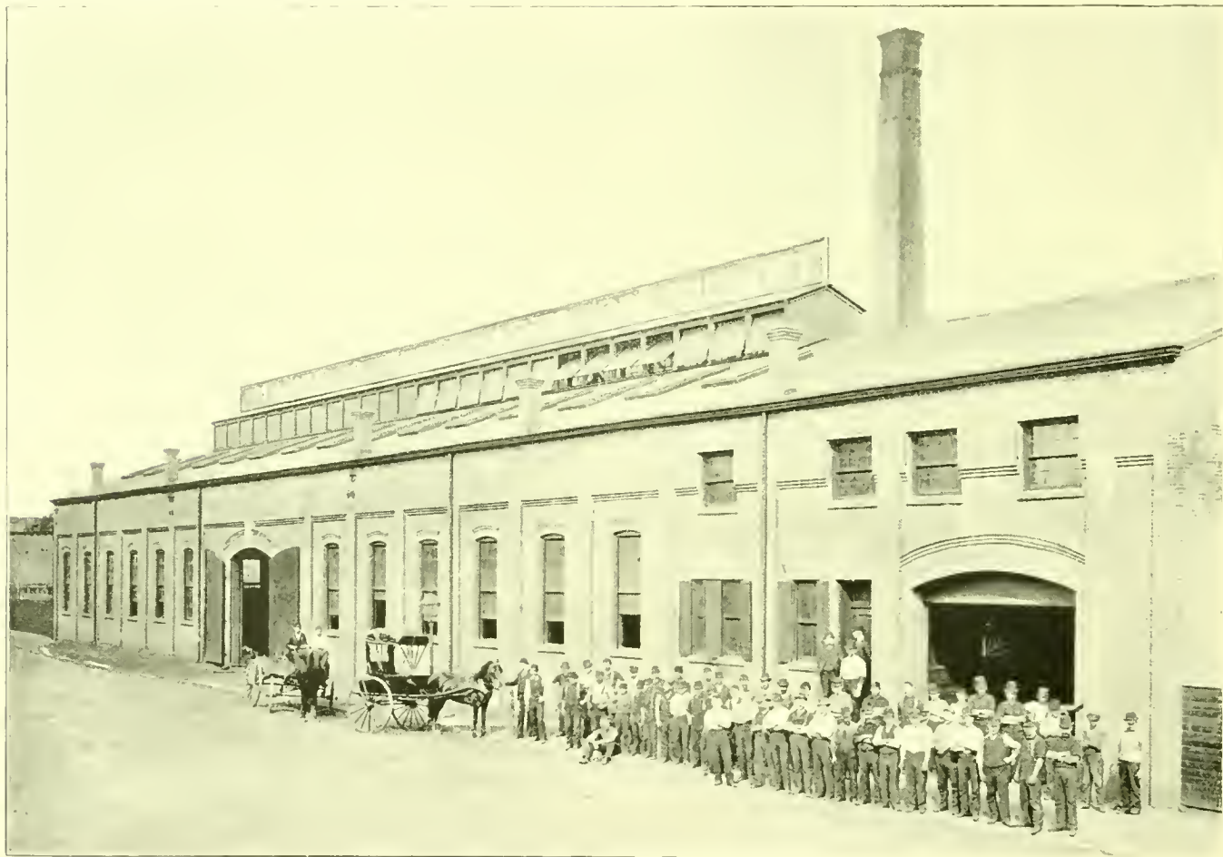
WORKS OF MAHER & FLOCKHART, ON POLK STREET.
