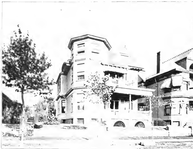
RESIDENCE OF A. J. GLASS, ON HUNTERDON STREET
