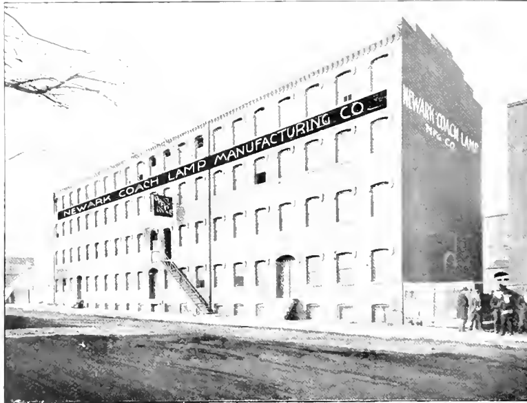
PLANT OF NEWARK COACH LAMP MANUFACTURING CO.
