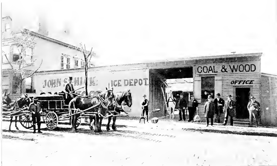
VIEW ON GARDEN STREET, SHOWING JOHN SCHICK'S COAL AND ICE DEPOT.
