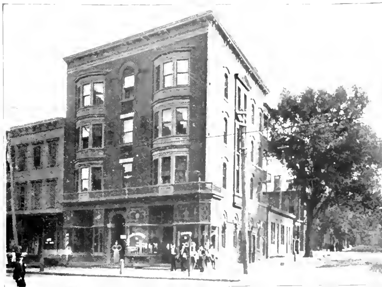
POORTMAN'S HALL, FERRY AND PROSPECT STREETS.
