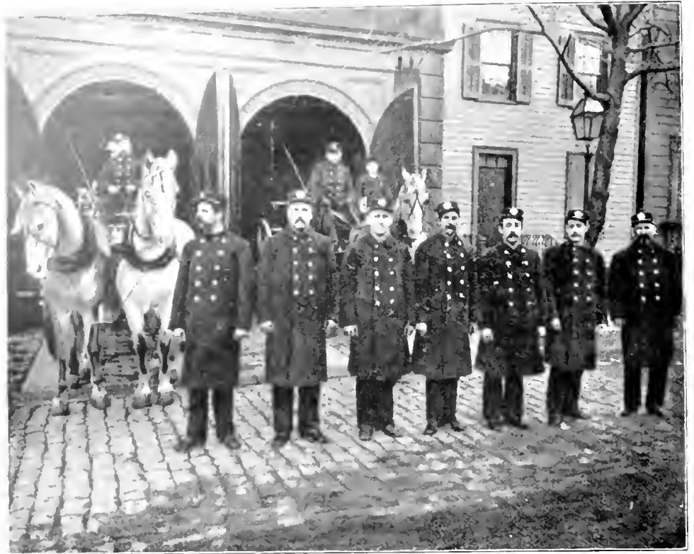
ENGINE COMPANY NO. 5, ON ESSEX STREET.
