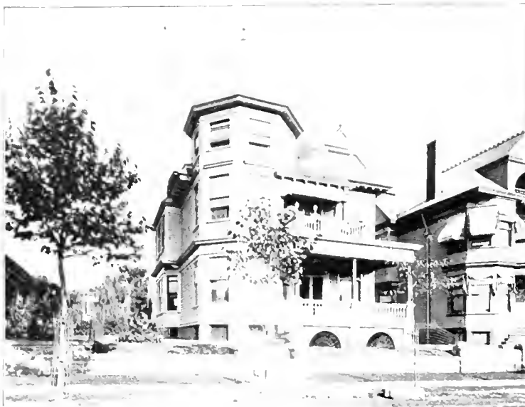
RESIDENCE OF A. J. GLISS, ON HUNTERDON STREET.
