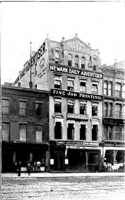
NEWARK DAILY ADVERTISER BUILDING.
