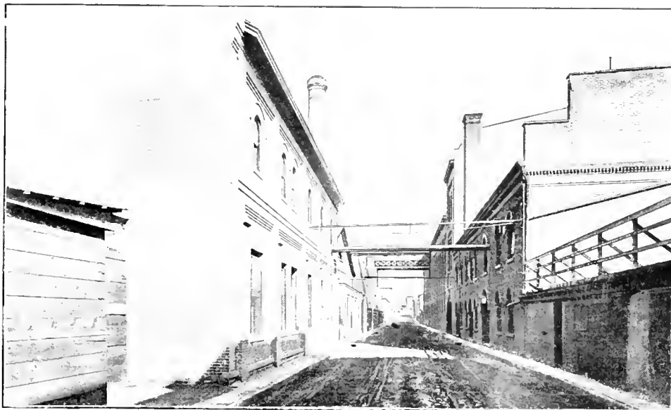
VIEW ON JERSEY STREET.
