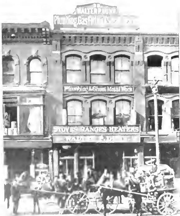
WALTER P. DUNN'S PLUMBING ESTABLISHMENT, 95 MARKET STREET, NEWARK, N. J.
