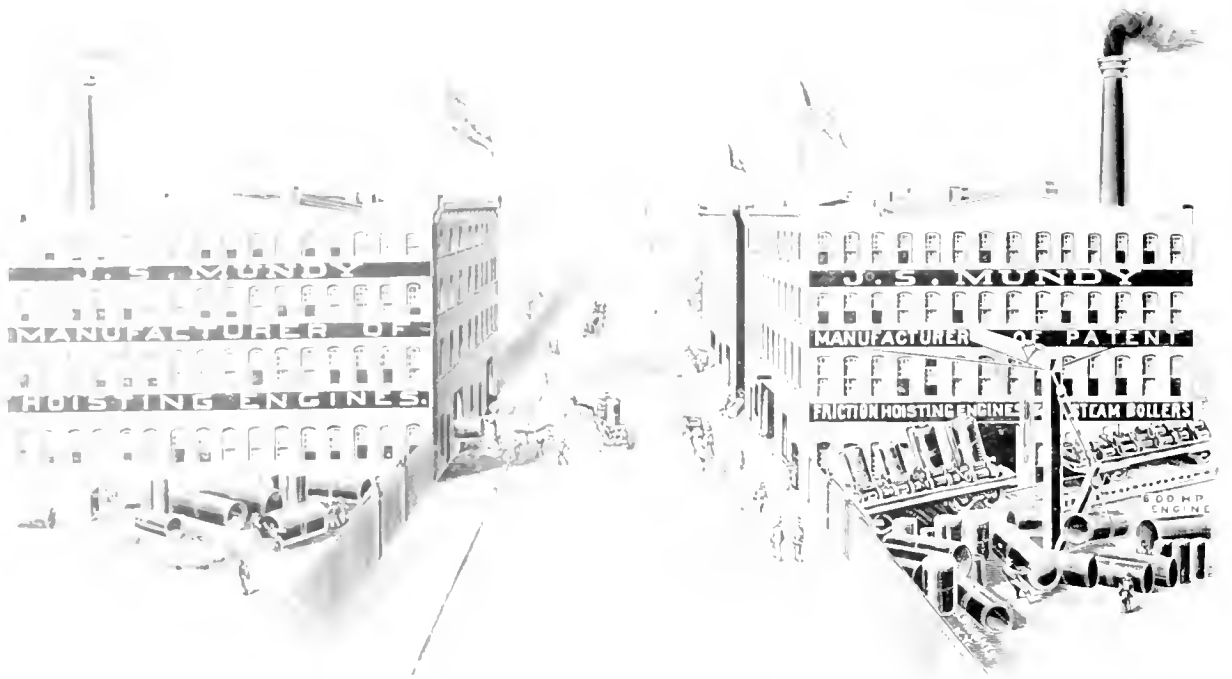
HOISTING ENGINES IN WORK ON ROBERT STREET.
