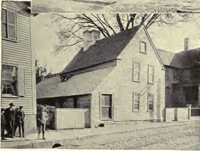
JOHN WARD HOUSE, Showing Overhanging Second Story and Corner Shop. NARBONNE HOUSE, Showing Lean-to Roof and Corner Shop.
