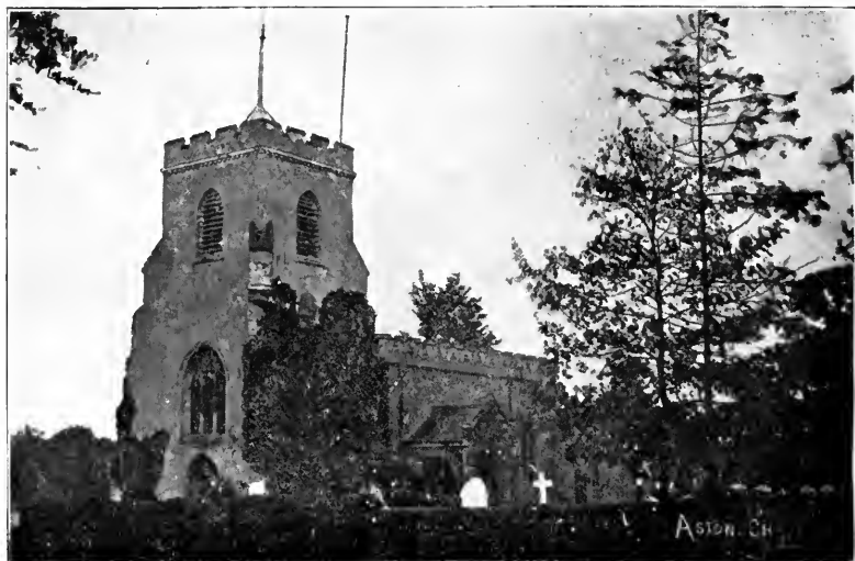
ASTON PARISH CHURCH, HERTFORDSHIRE, ENGLAND
