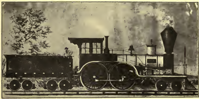
LOCOMOTIVE "LAWRENCE," WEIGHT TWENTY-FIVE TONS Built by the Lawrence Machine Shop, 1853
