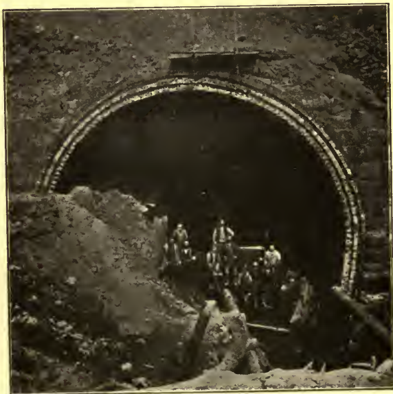
HOOSAC TUNNEL UNDER CONSTRUCTION, 1871
