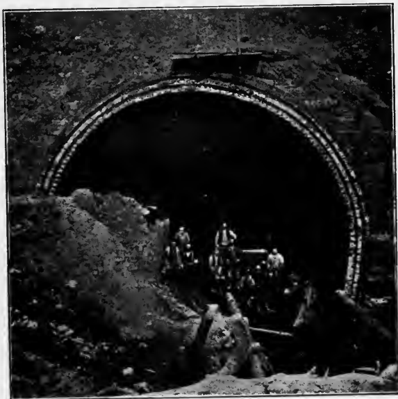
HOOSAC TUNNEL UNDER CONSTRUCTION, 1871
