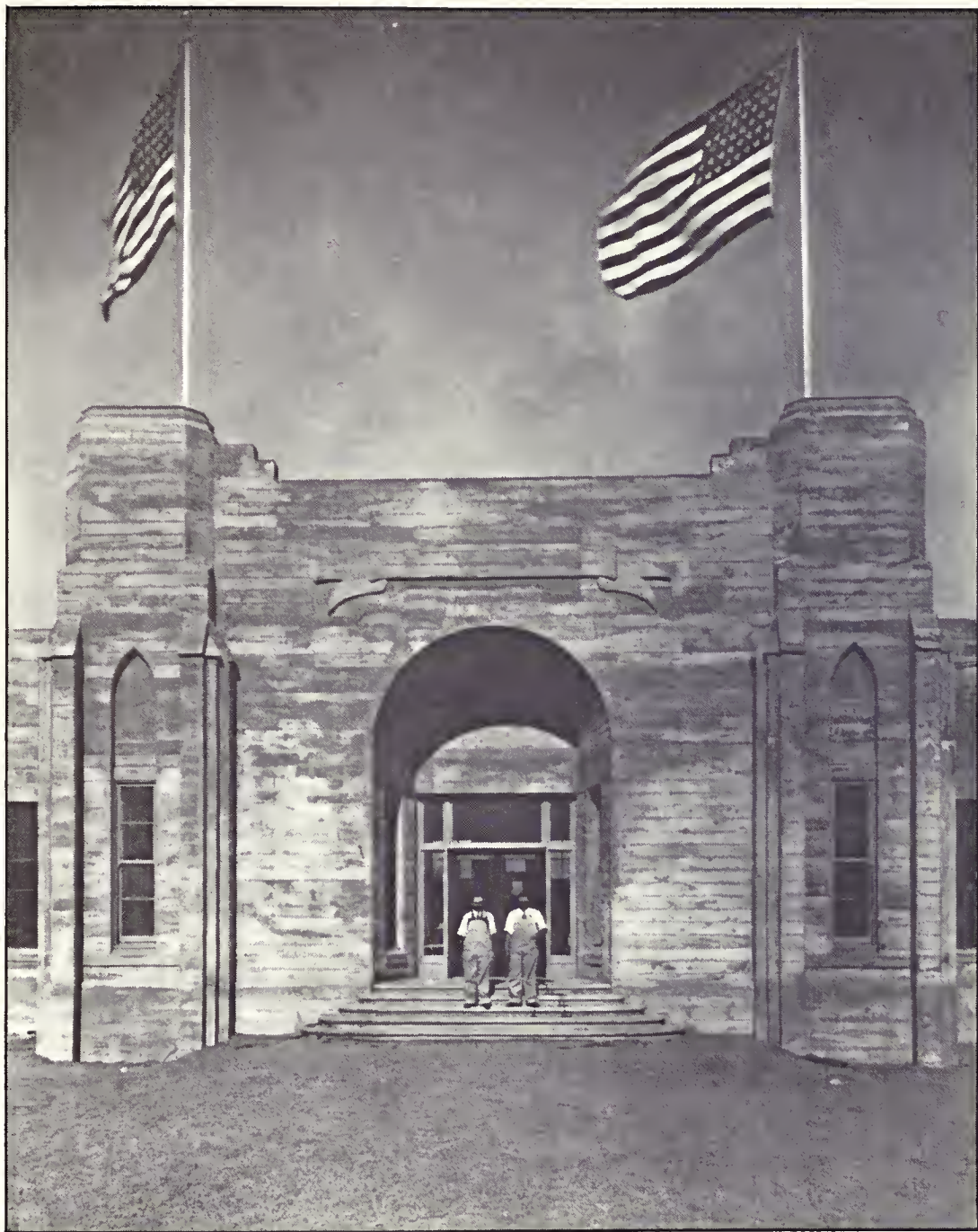
Main entrance to offices at Filice & Perrelli plant, Richmond, 1930.
