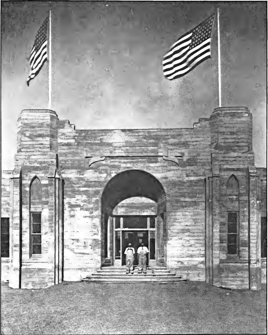
Main entrance to offices at Filice & Perrelli plant, Richmond, 1930.
