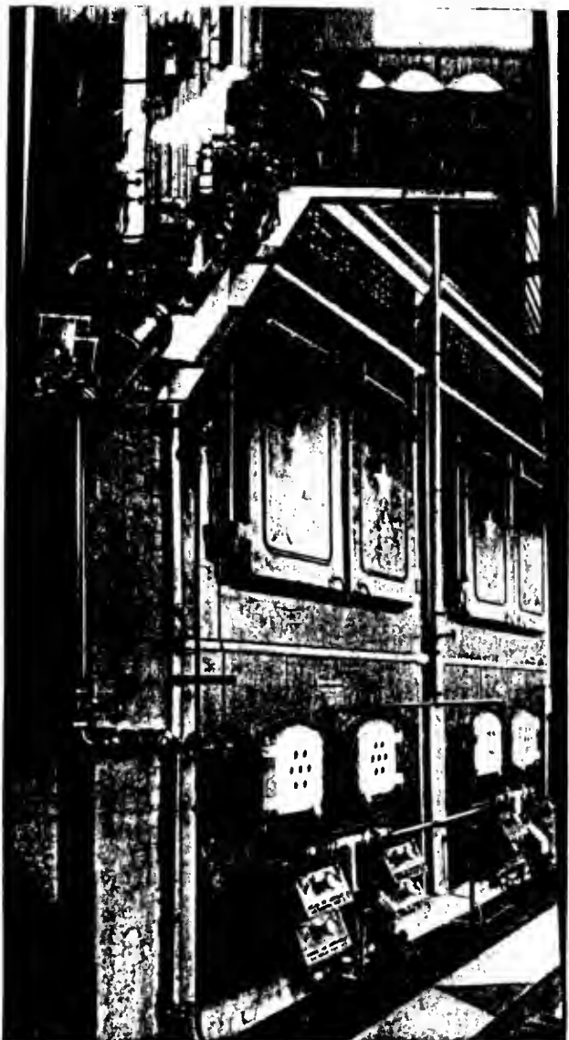
Above—Pumping system and lubricating oil storage service tanks in gas-fired 1000 hp. steam boiler plant.
