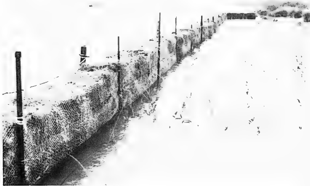
Figure 9. A temporary wave-stilling device constructed in Block IX. The device is constructed of pipe, wire netting, cable, and baled hay.
