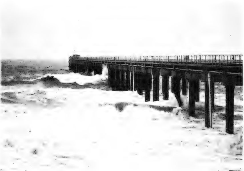
Figure 8. Waves at the FRF on 13 September 1978. Note waves breaking on the piles.
