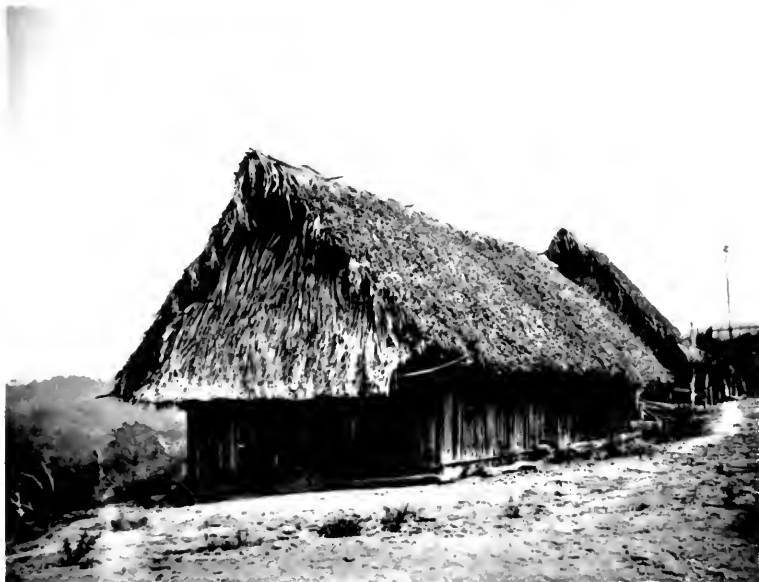
2. END VIEW OF HOUSE, SAN ANTONIO (p. 91)
