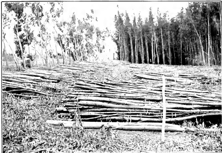
A. LOGS READY TO BE CUT BY STEAM SAWING MACHINE. VISIBLE IN BACKGROUND.
