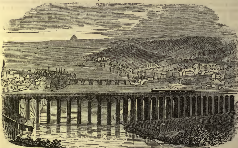
Viaduct and Bridge across the Tweed.
