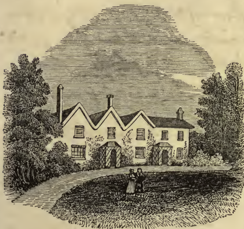
Moore's Cottage, Sloperton.
