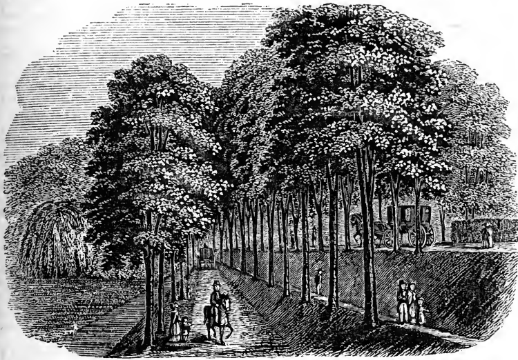
Dyke between Rotterdam and Delftshaven.
