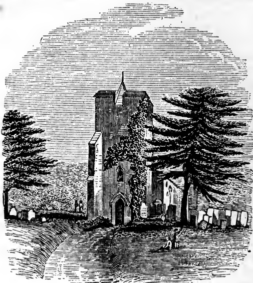
St. Martin's Church, near Canterbury.
