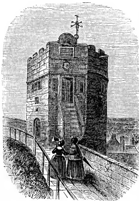
Phoenix Tower, Chester.
