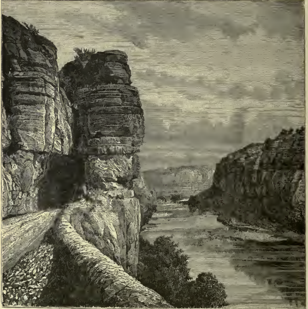
Fig 134.--THE DEFILE OF THE ARDÈCHE, NEAR ROOMS.
