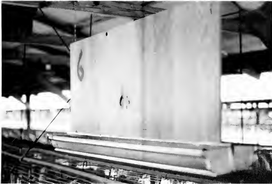
Figure 7. Panel with guttering suspended by chains at the tilling site.
