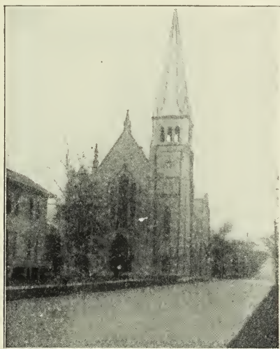
FIRST METHODIST EPISCOPAL CHURCH COMPLETED IN 1872
