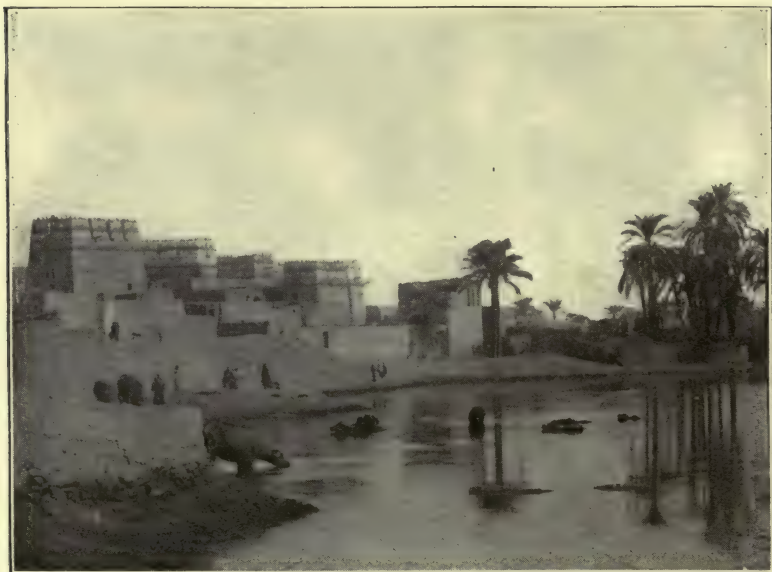
SCENE IN EGYPT, WHICH IS IN THE SAME LATITUDE AS SOUTH FLORIDA, WHERE FLAT ROOFS NOT ONLY PREVAIL, BUT WHERE THEY ARE USED AS MUCH AS ANY ROOM IN THE DWELLING.
