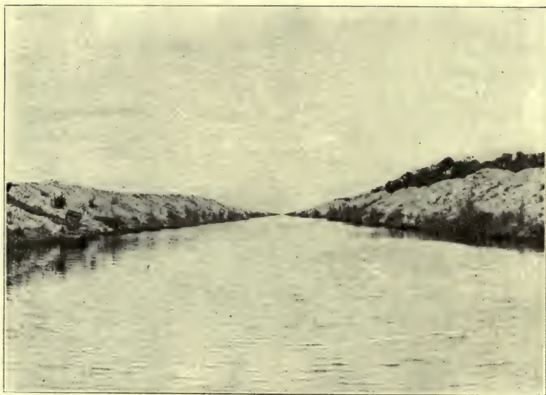
STATE CANAL IN THE EVERGLADES, FOR DRAINAGE, IRRIGATION AND TRANSPORTATION.
