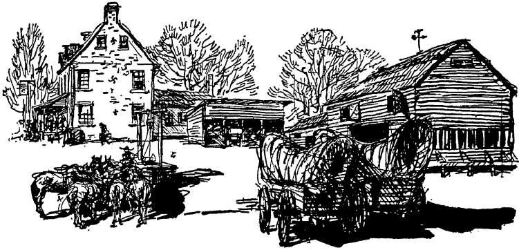
Stagehouse on the National Road
