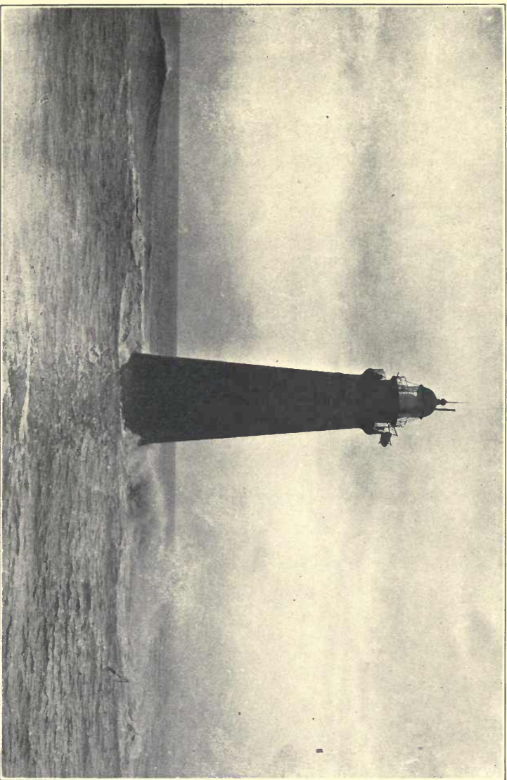
A SILENT HELPER IN DEEP WATERS MINOT'S LEDGE LIGHT STATION, MASSACHUSETTS
