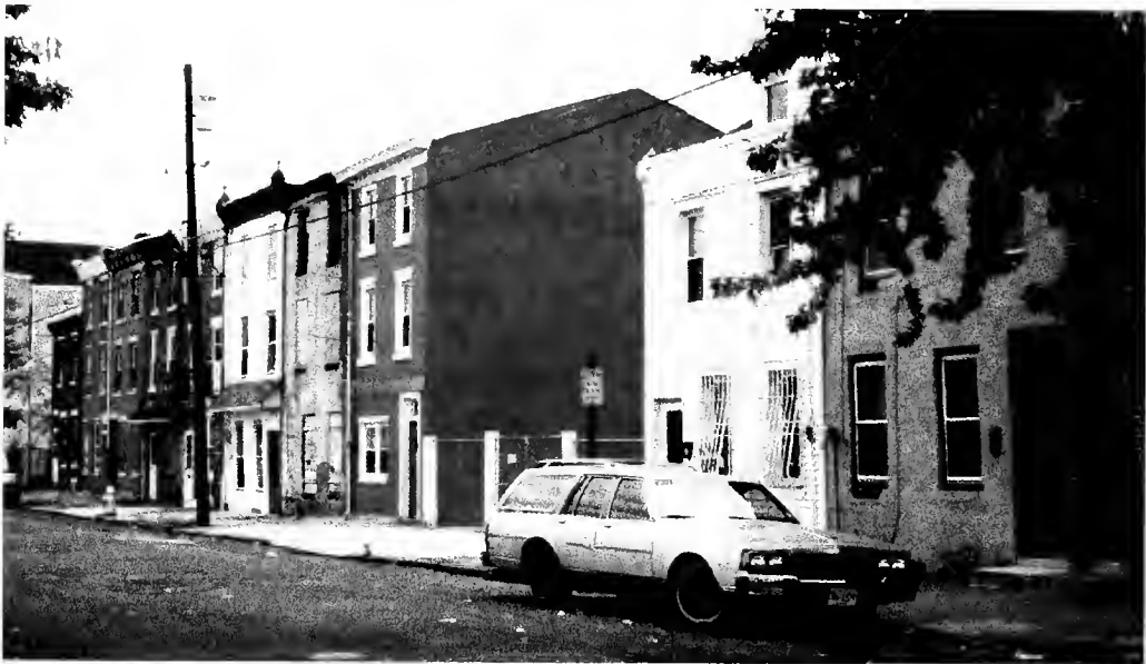
Figure 15: Streetscape showing facade alterations.
