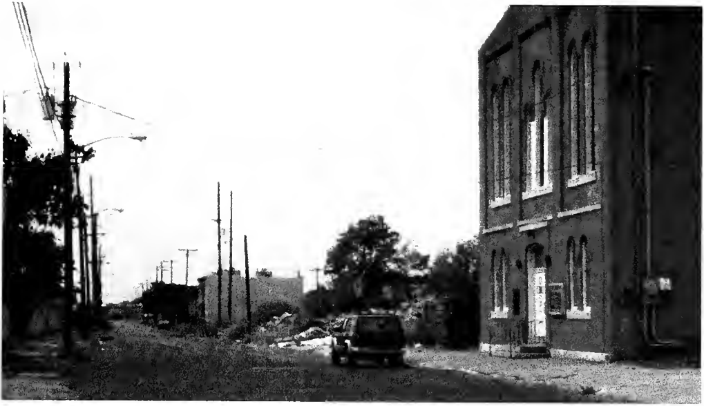
Figure 14: View of Macedonia AME Church and adjacent rubble looking west.
