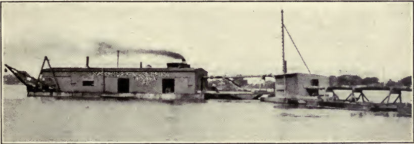
FIG. 2.—HYDRAULIC DREDGE BUILDING LEVEE.
