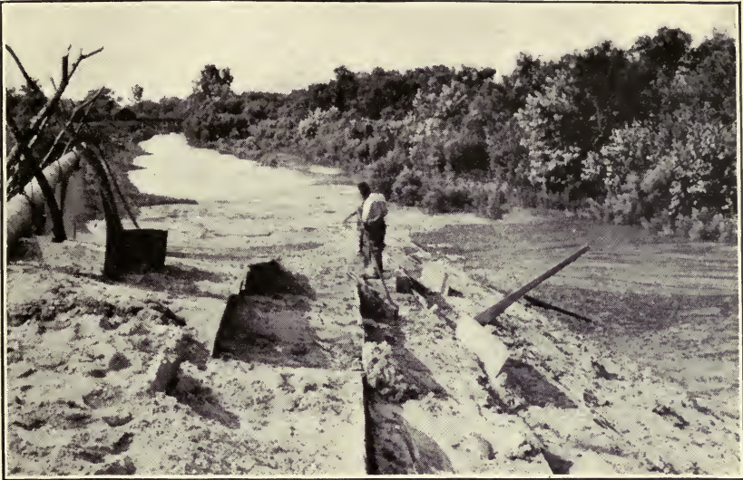
FIG. 1.—BUILDING A LEVEE BY MEANS OF STAGGERED SLOPE BOARDS.
