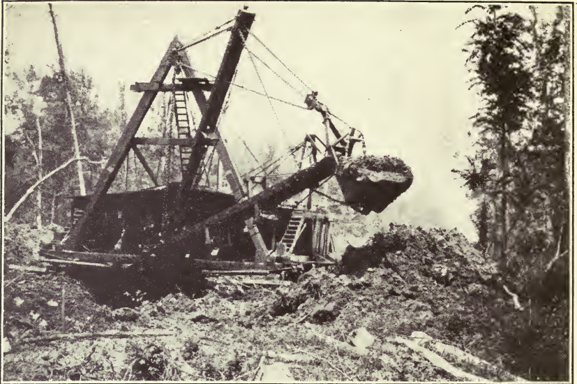
FIG. 1.—WALKING DRY-LAND DIPPER DREDGE WITH DOUBLE BOOM AND SCOOP BUCKET.
