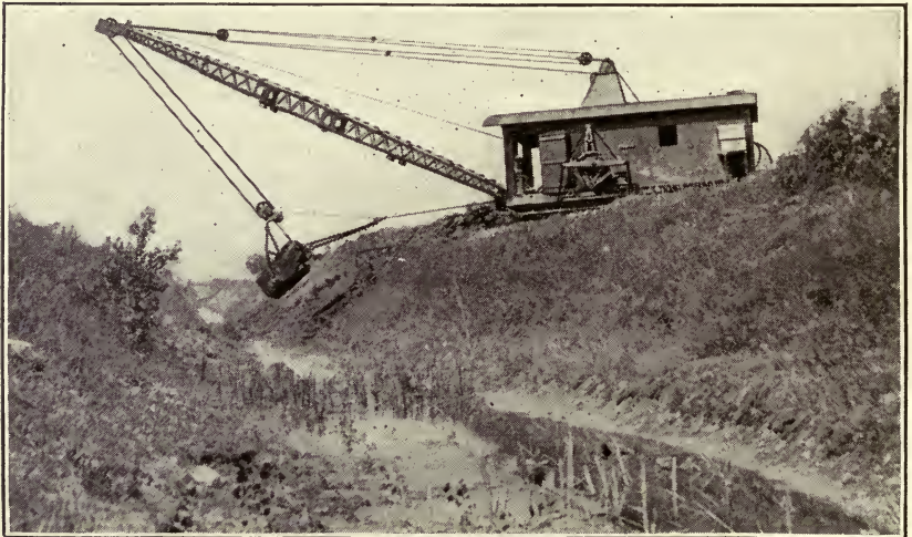
FIG. 2.—ENLARGING AN OLD DITCH BY ROTARY DRAG LINE EXCAVATOR WORKING FROM BANK.
