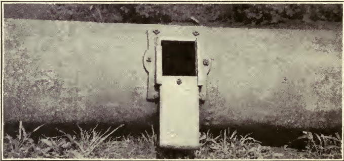
FIG. 2.—DISCHARGE PIPE OPENING WITH SHUTTER.
