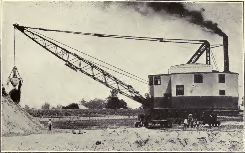
FIG. 1.—DRY-LAND ROTARY GRAB-BUCKET EXCAVATOR.
