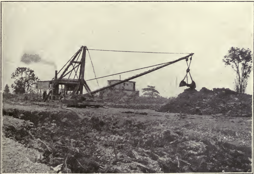
FIG. 2.—NONROTATING DRY-LAND GRAB-BUCKET EXCAVATOR.
