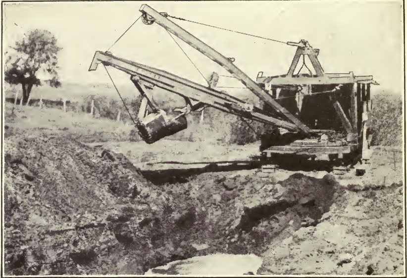
FIG. 1.—NONROTATING SCRAPER EXCAVATOR WITH SLIDING TRACK MOUNTING.
