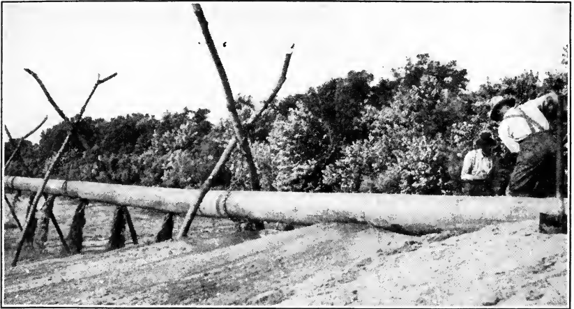
FIG. 1.—DISCHARGE PIPE OF HYDRAULIC DREDGE SHOWING MATERIAL PASSING THROUGH OPENINGS IN BOTTOM OF PIPE.
