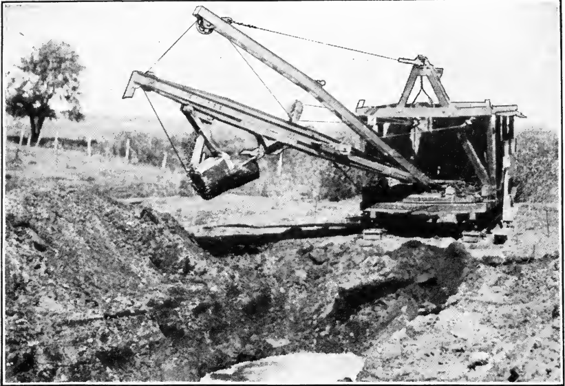
FIG. 1.—NONROTATING SCRAPER EXCAVATOR WITH SLIDING TRACK MOUNTING.
