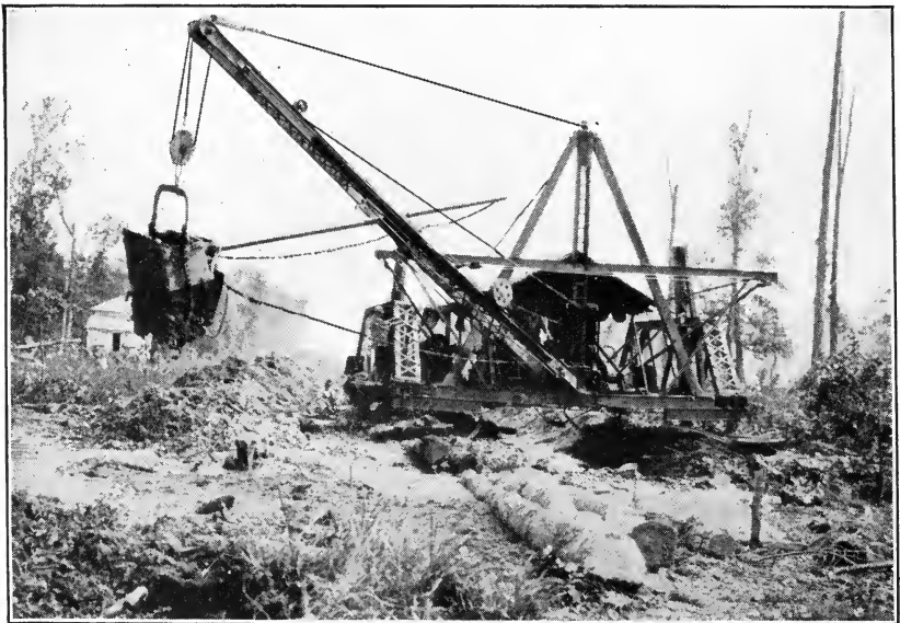
FIG. 2.—WALKING DRY-LAND DIPPER DREDGE.
