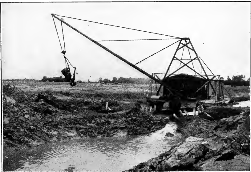
FIG. 2.—NONROTATING TYPE OF DRAG-LINE EXCAVATOR WITH WHEEL MOUNTING.
