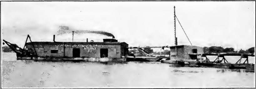
FIG. 2.—HYDRAULIC DREDGE BUILDING LEVEE.
