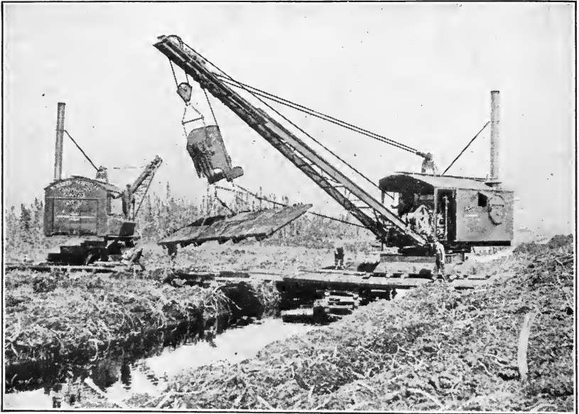
FIG. 1.—DRAG-LINE EXCAVATOR ON SKID-AND-ROLLER MOUNTING TRANSFERRING A SECTION OF TRACK AHEAD.
