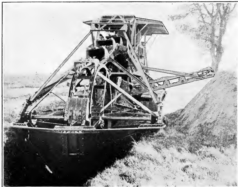
FIG. 2.—CONVERTIBLE TYPE OF WHEEL EXCAVATOR.
