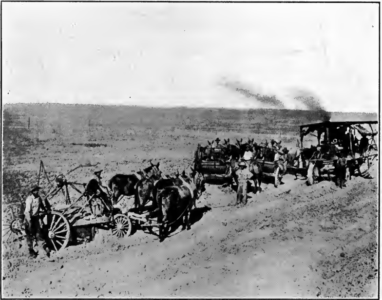
FIG. 158.—Maney scrapers on irrigation work. (Courtesy of Baker Mfg. Co.)
