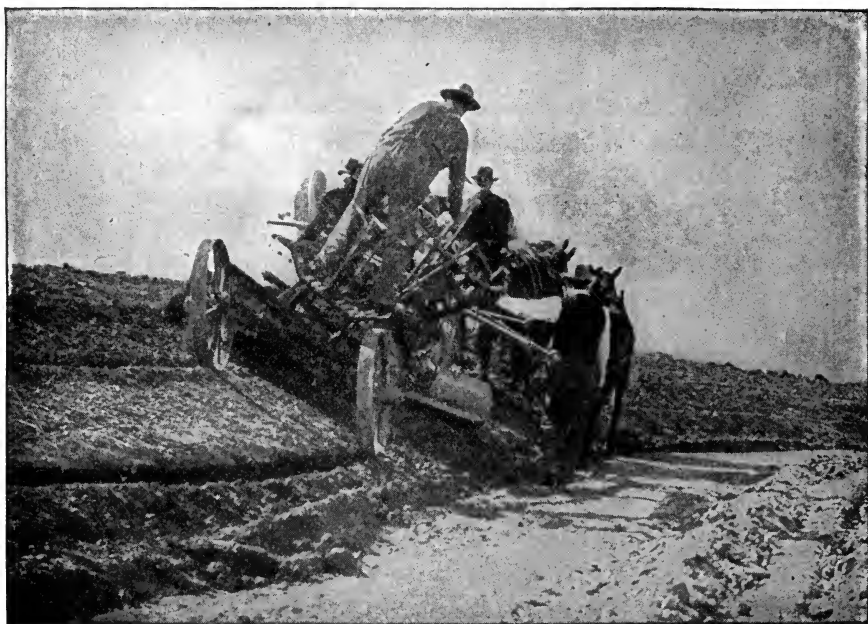
FIG. 15.—Reclamation grader excavating irrigation ditch.
