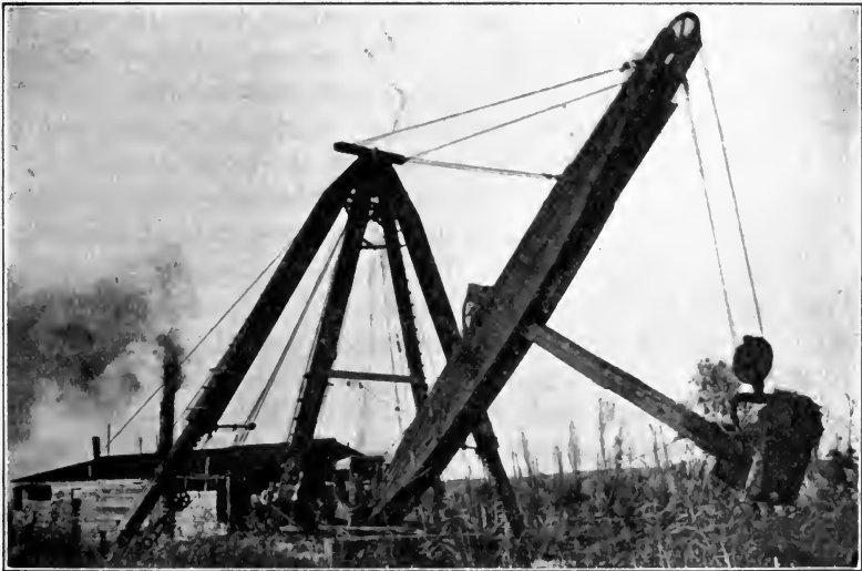
FIG. 99.—Dipper dredge with bank spuds excavating drainage ditch. (Photo by Author.)
