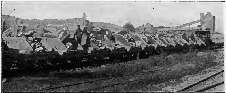
FIG. 194.—Loaded skips on way to crusher. ( Compliments of Edison Portland Cement Co. )
