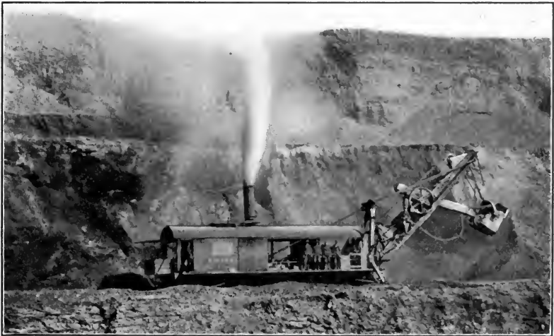
FIG. 199.—Steam shovel excavating iron ore in Minnesota. (Courtesy of The Bucyrus Co.)
