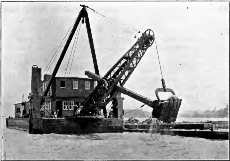
FIG. 174.—Dipper dredge constructing harbor channel.
