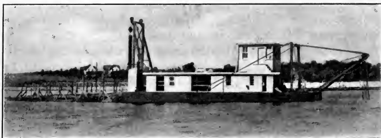
Fig. 176.—Electrically operated hydraulic dredge on lake improvement. (Courtesy of Norbom Engineering Co.)
