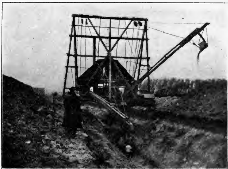
FIG. 34.—Traction excavator with two booms.
