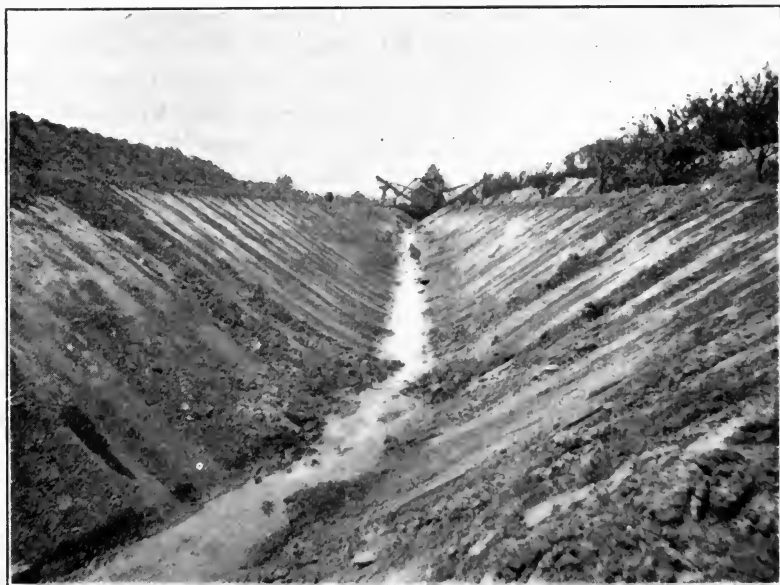
FIG. 163.—Templet excavator constructing irrigation ditch. (Courtesy of F. C. Austin Co.)
