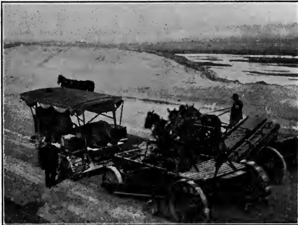
FIG. 160.—Elevating grader on canal construction.
