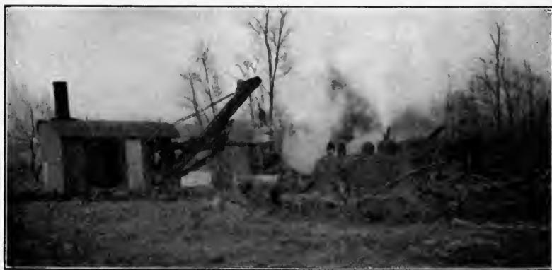
FIG. 189.—Revolving shovel loading train with clay. (Photo by Author.)
