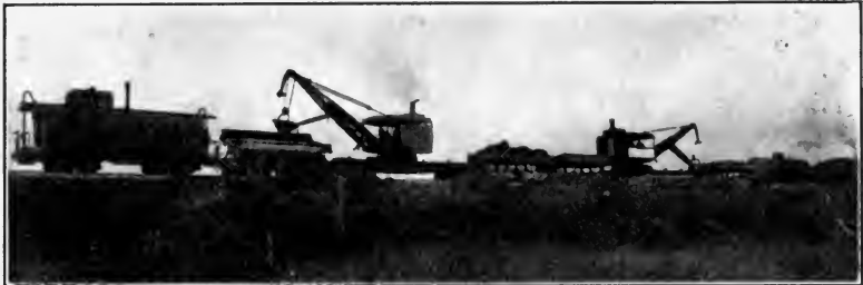
FIG. 156.—Double ditcher railway train. (Courtesy of American Hoist & Derrick Co.)
