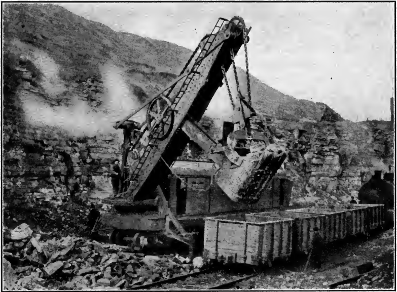
FIG. 196.—Steam shovel loading train of box cars.
