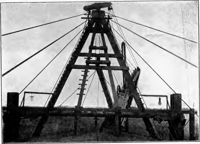
FIG. 93.—A-frame of floating dipper dredge. (Photo by Author.)
