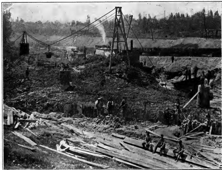
FIG. 86.—Cableway excavator digging a sewer trench.
