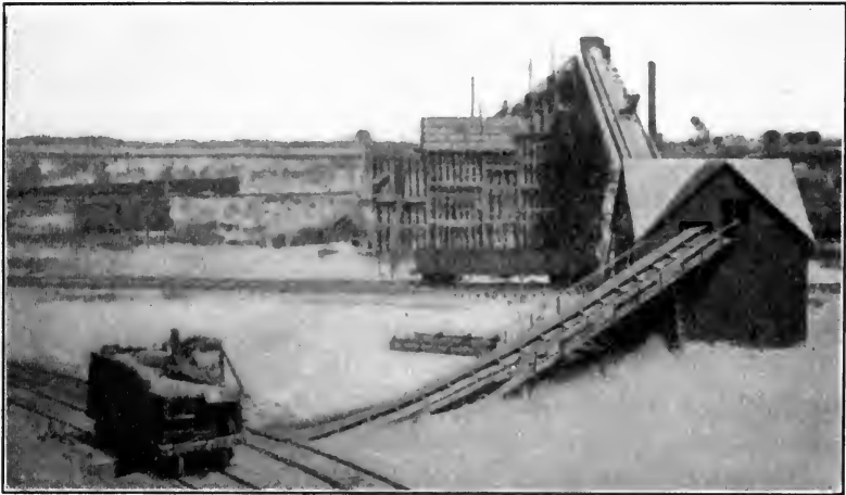
FIG. 204.—Hopper car discharging on to belt conveyor at a sand plant. (Courtesy of The Excavating Engineer .)
