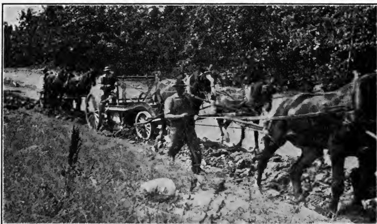
FIG. 130.—Four-wheel scrapers on highway construction.
