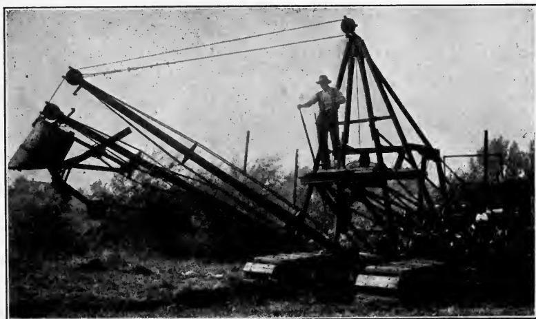
FIG. 35.—Gopher dry-land traction ditcher. (Courtesy of Dix Machine Co.)
