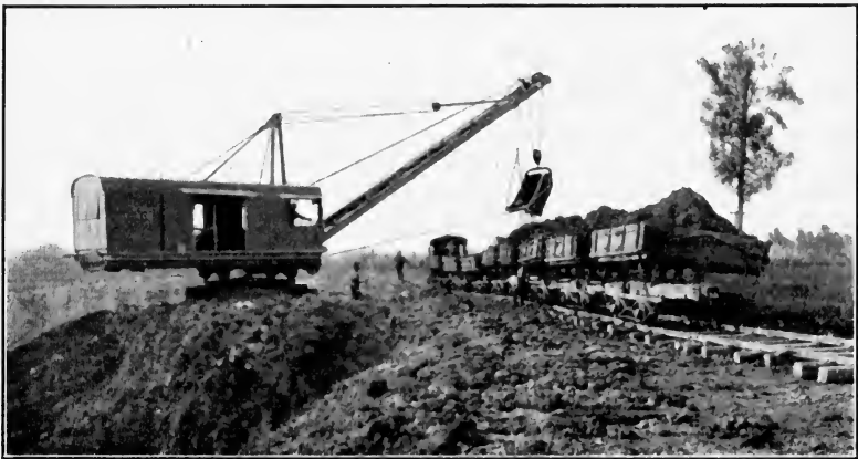
FIG. 205.—Drag-line excavator operating clay pit. (Courtesy of The Excavating Engineer. )
