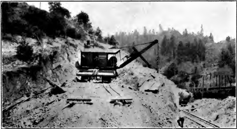
FIG. 138.—Revolving shovel on highway construction. (Courtesy of the Excavating Engineer.)
