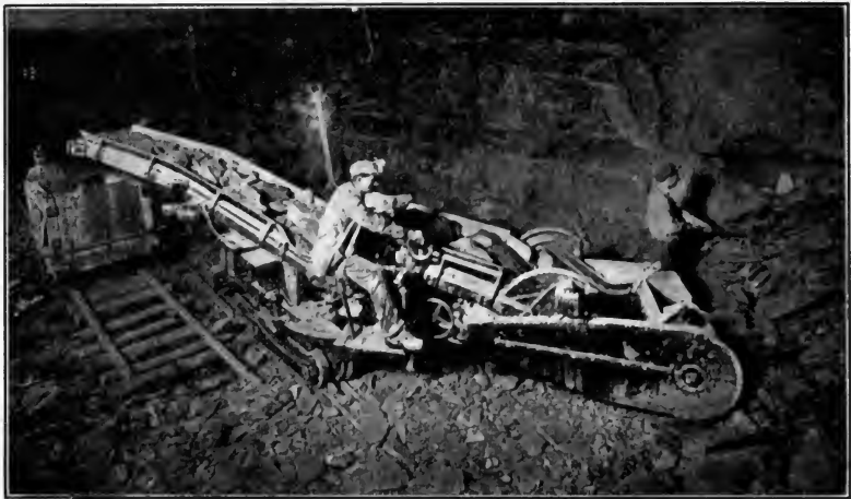
FIG. 209.—Shoveling machine operating in a coal mine. (Courtesy of Myers-Whaley Co.)
