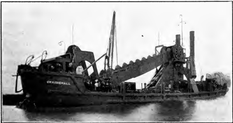
FIG. 103.—A deep-water ladder dredge.
