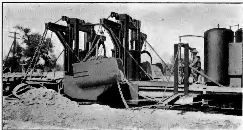
FIG. 157.—Bowman ditcher on railroad maintenance.
