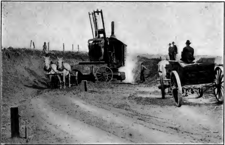
FIG. 139.—Highway construction in rolling country. (Courtesy of the Excavating Engineer.)
