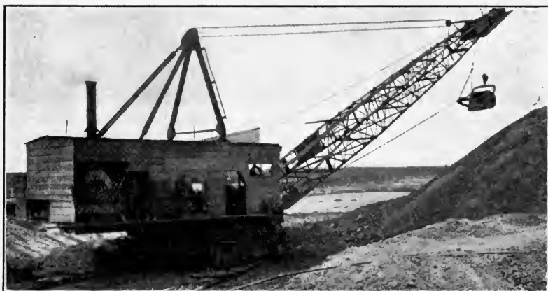
FIG. 151.—Drag-line excavator on railroad construction. (Courtesy of The Excavating Engineer.)
