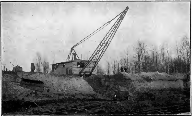
FIG. 190.—Scraper-bucket excavator stripping quarry.
