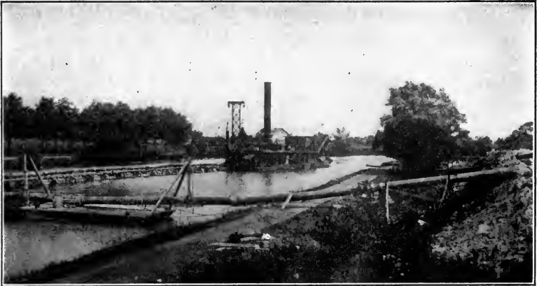
FIG. 114.—Discharge pipe of hydraulic dredge. (Courtesy of N. Y. State Engineer.)
