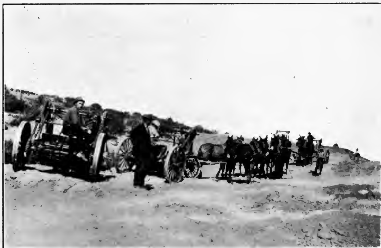
FIG. 145.—Maney scrapers on railroad construction. (Courtesy of Baker Mfg. Co.)
