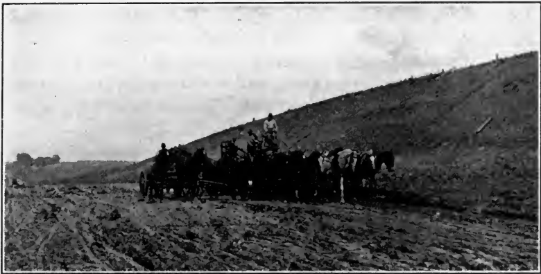
FIG. 147.—Elevating grader on railroad construction.
