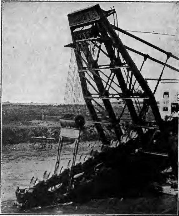
FIG. 104.—Bucket chain and gantry of ladder dredge.
