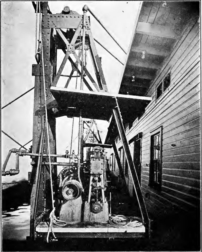
FIG. 121.—Side view of drill frame and engine. (Courtesy of Ingersoll-Rand Co.)
