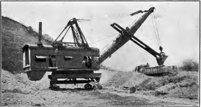
FIG. 203.—Large revolving shovel operating gravel pit. (Courtesy of The Excavating Engineer .)
