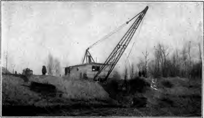
FIG. 47.—Drag-line excavator with steel framed boom.
