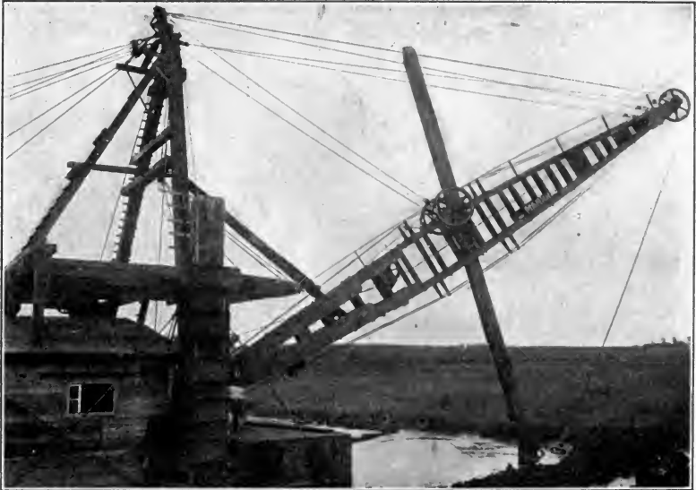
FIG. 97.—Boom and dipper handle of floating dipper dredge. (Photo by Author.)
