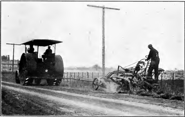
FIG. 133.—Blade grader shaping-up earth road. (Photo by Author.)
