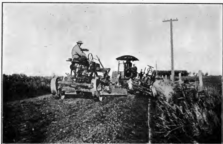
FIG. 134.—Reclamation graders on road construction.
