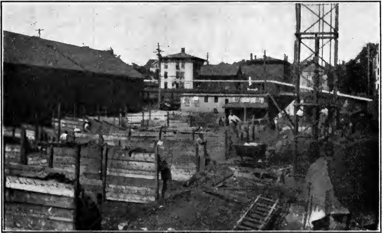
FIG. 185.—View of bulkhead method of footing pit excavation. (Photo by Author.)
