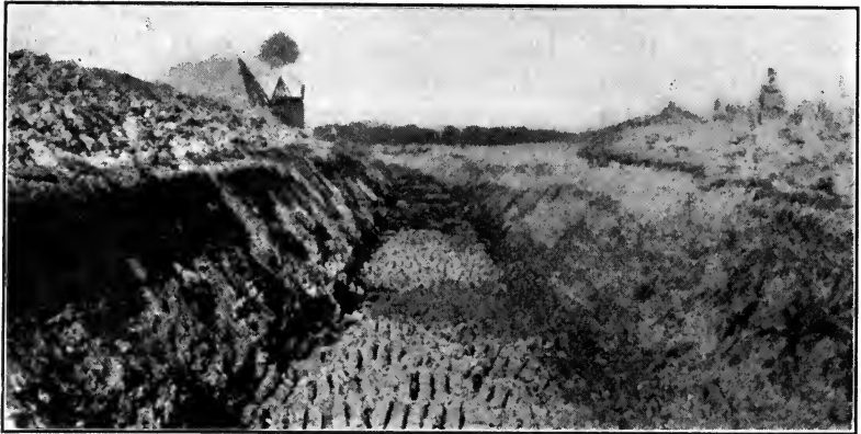
FIG. 152.—Railroad cut made by drag-line excavator. (Courtesy of The Excavating Engineer. )
