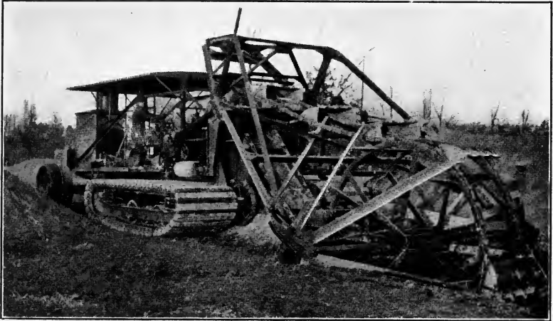
FIG. 77.—Wheel excavator constructing small ditch. (Courtesy of F. C. Austin Co.)
