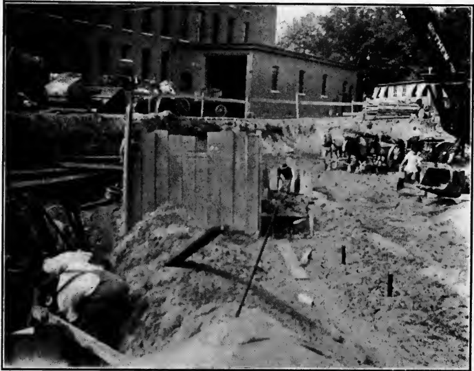
FIG. 187.—Levelling-up basement excavation with scraper. (Photo by Author.)
