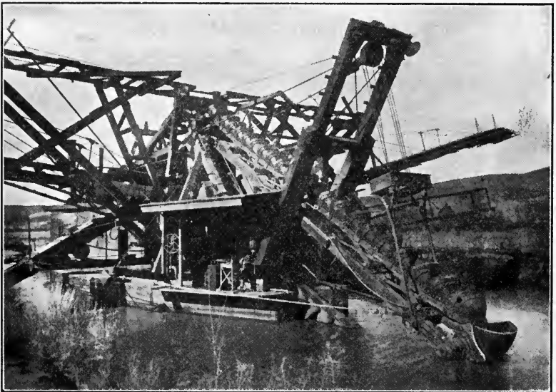
FIG. 108.—Ladder dredge excavating irrigation canal. (Courtesy of the Reclamation Service.)
