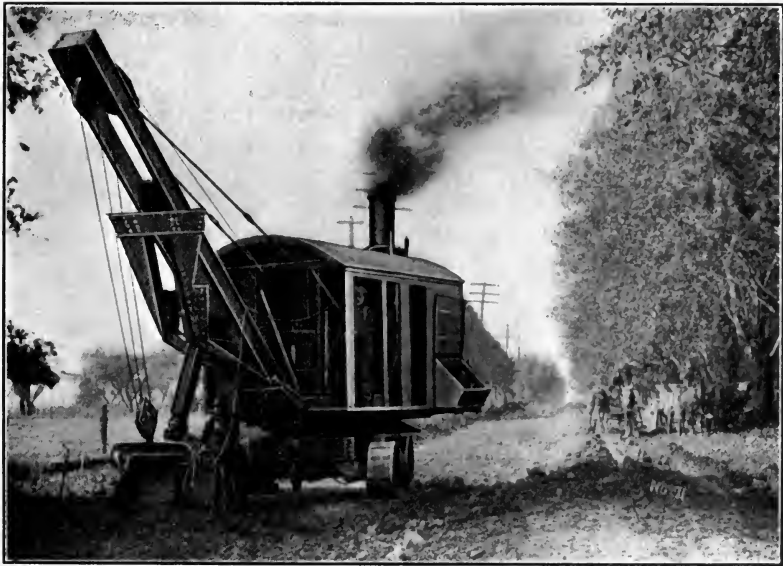
FIG. 140.—Steam shovel excavating for pavement. (Courtesy of Thew Automatic Shovel Co.)
