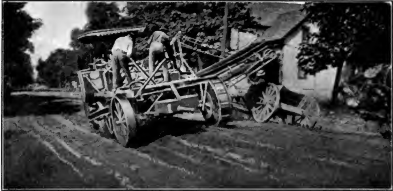
FIG. 136.—Elevating grader on road construction. (Courtesy of Western Wheeled Scraper Co.)
