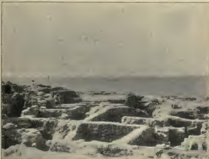
FIG. 11. —THE EXCAVATED PART OF THE SITE LOOKING TOWARDS THE S. END OF THE PALACE.
