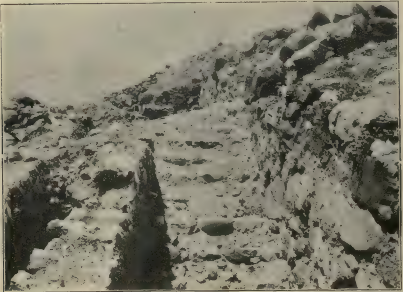
FIG. 18. VIEW OF STAIRCASE. (Partly obliterated by debris fallen since excavation.)
