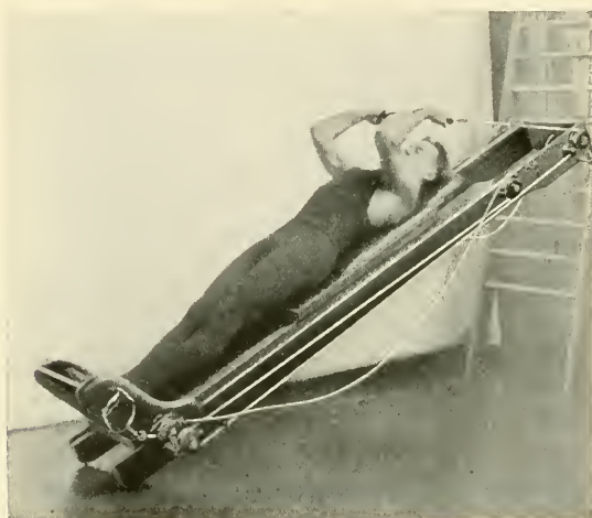
Fig. 32.—Goldie's exerciser in use. By grasping the handles beside the feet a change in action is obtained. One upper and one lower handle may also be used together, and the resistance increased by hooking the frame to a higher rung (Spalding).
