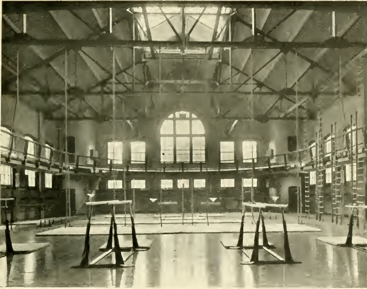
Fig. 114.—The main exercise hall of the Brookline municipal gymnasium and baths.
